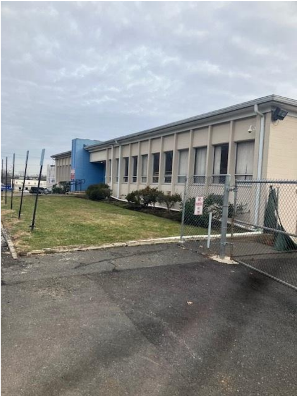
PHOTO 2 FACING ALONG LOT 10 ( 29 River Rd)
