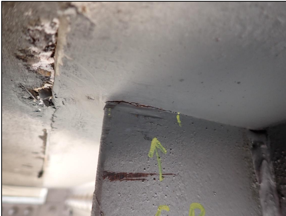
Figure 11: SA Cracked Tack Weld – Girder B South Face – Stiffener 17 to Horizontal Leg of Top Flange Angle
