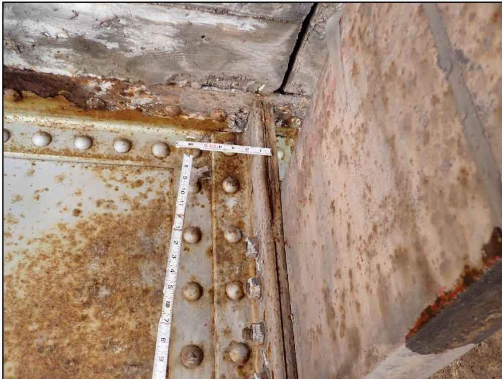
Figure 27: Typ. Pack Rust between Bearing Stiffeners of Int. Girders at Pier – Girder E S. Face at P4 – Stiffener 69
