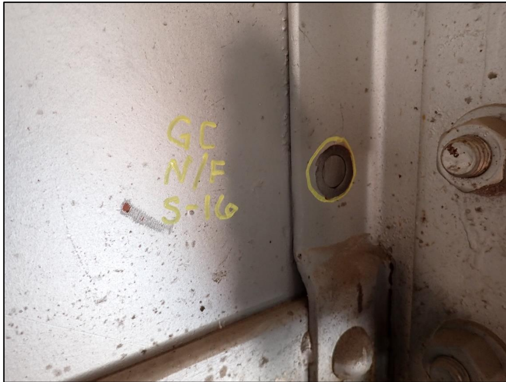
Figure 23: Sheared Rivet Head – Girder C North Face at Stiffener 16 Near Bottom
