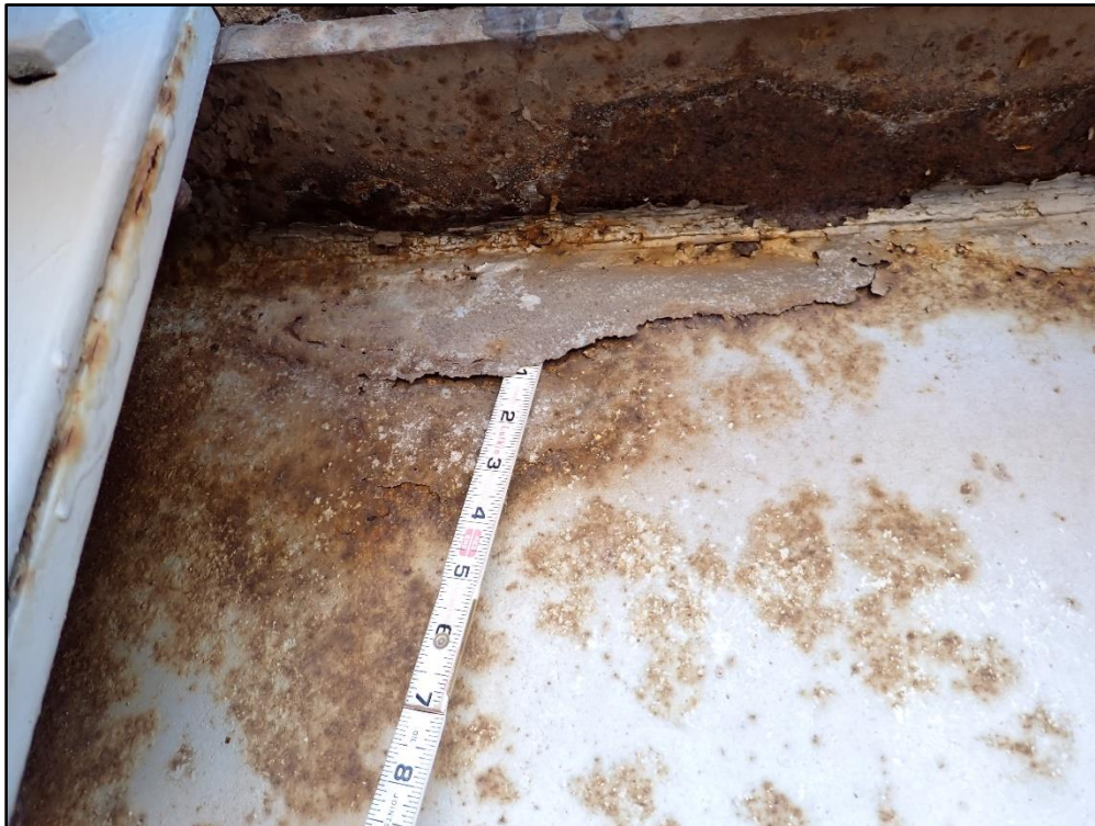
Figure 31: Laminar Corrosion in Top of Web of North Exterior Girder A
