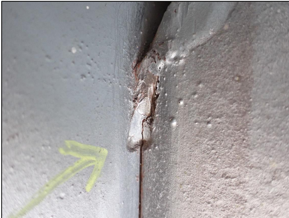
Figure 17: NSA Cracked Tack Weld – Girder E South Face – Stiffener 55 to Web
