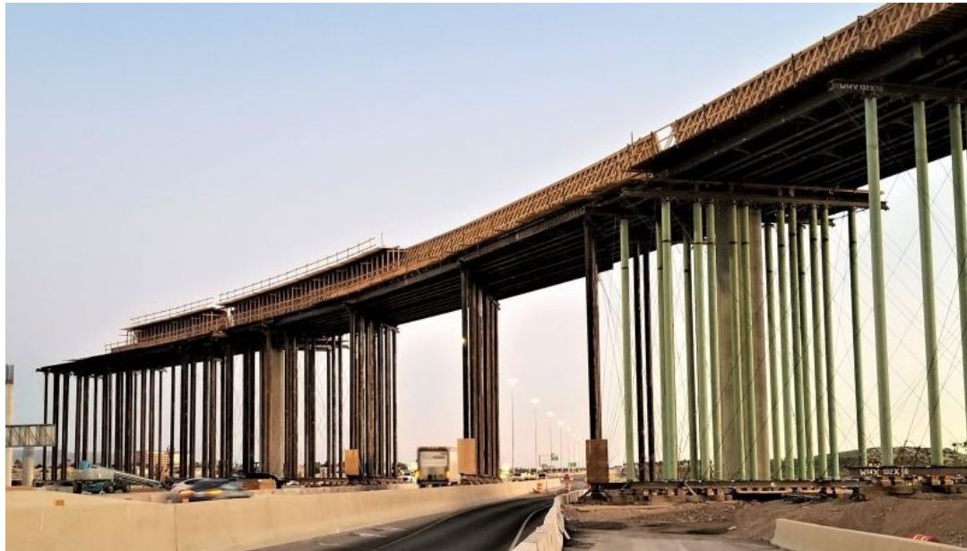
Figure 38. Example Falsework Photo for Cast-in-place Concrete Construction
