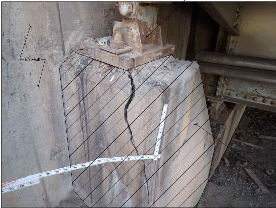
ABUTMENT 6-SUPPORT PEDESTAL AT GIRDER "A"
