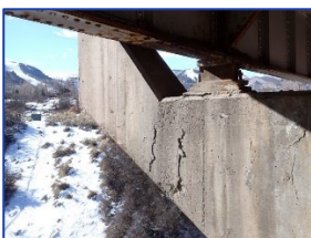
Light scale cracking typical at all pier caps
