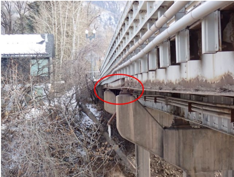
Figure 15. Girder F Sagging Near Mid-span
