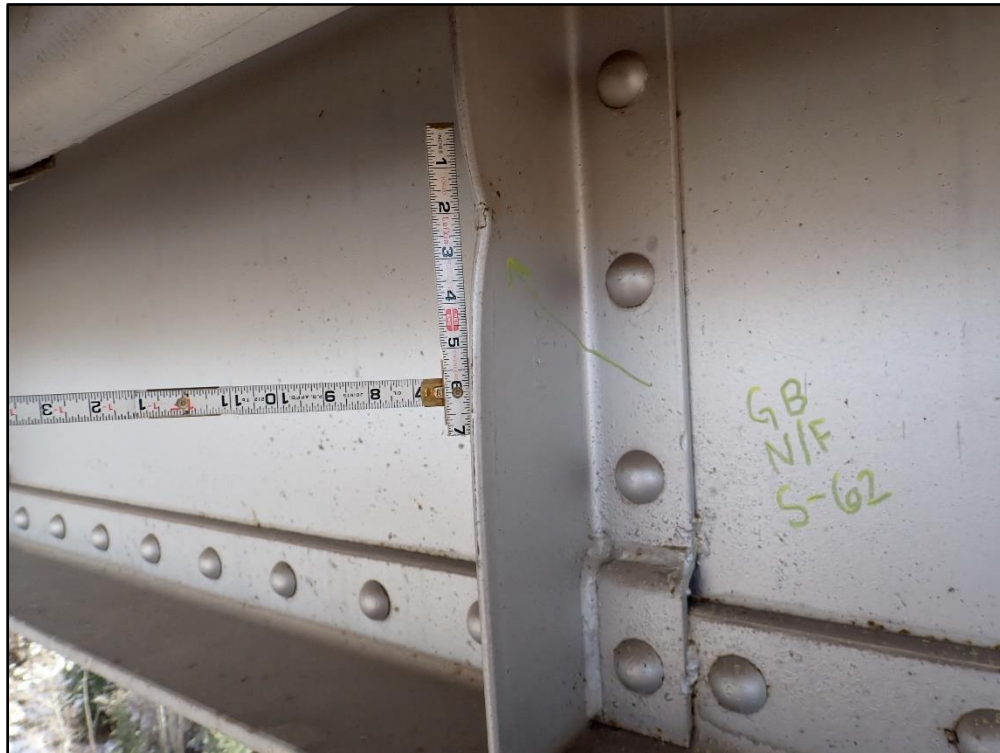
Figure 29: Deflection of Stiffener 62 at North Face of Girder B
