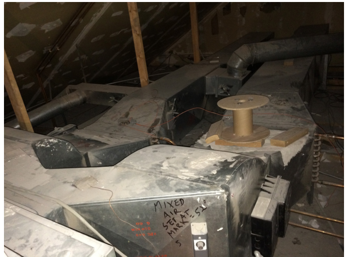
Two-Zone Reheat System with Uninsulated Ducts
