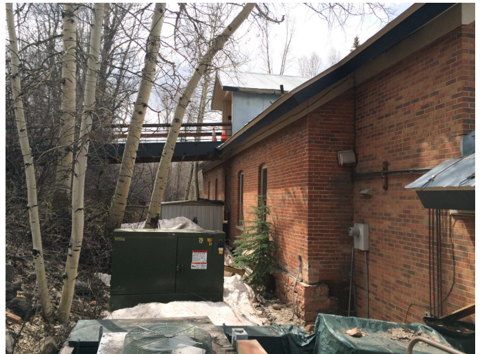
Exterior transformer exposed to potential ice damage
