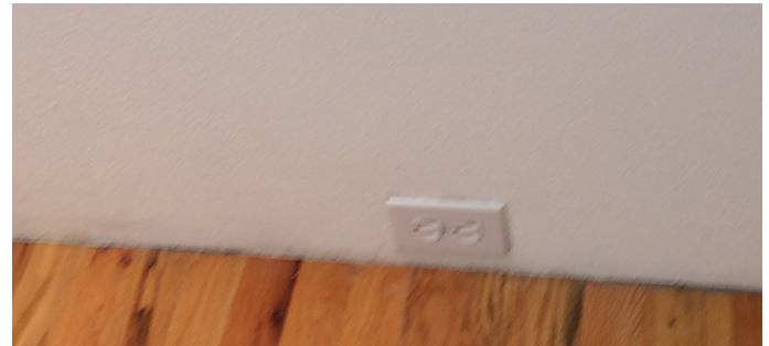
Receptacles at art display areas mounted unusually low
