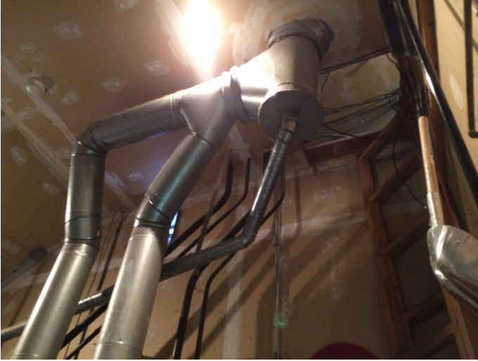
Common Venting Through Mech Room Ceiling
