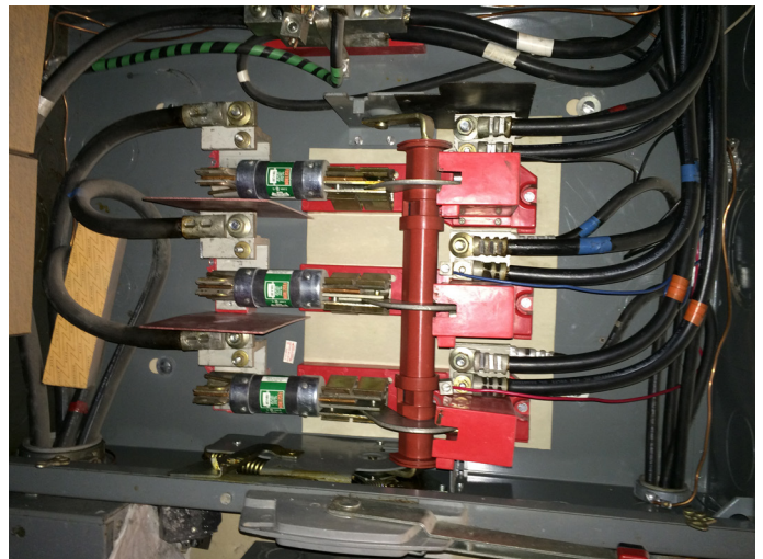
Interior Incoming service and main disconnect
