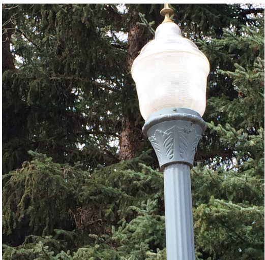
Acorn style pole mounted area lighting at parking
