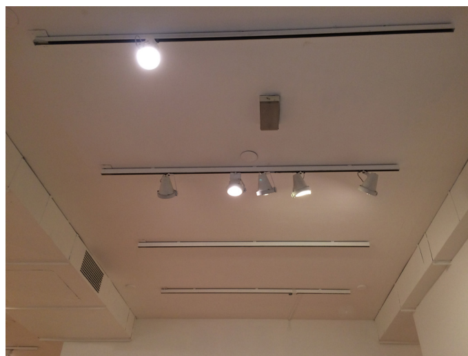
Specialty incandescent/halogen track lighting throughout the art display area
