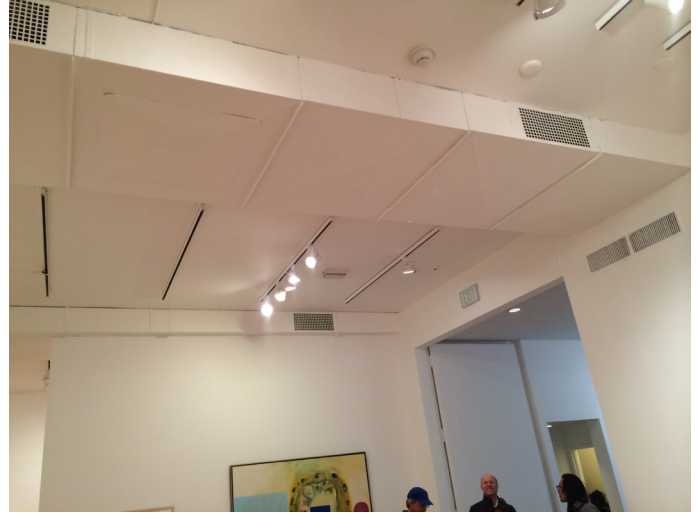
Ducting and Diffusers in Lower Gallery
