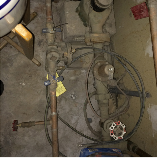
1½" Water Entry Assembly (PRV, BFP, Meter)
