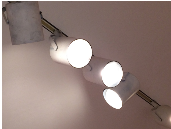
Specialty incandescent/halogen track lighting throughout the art display area
