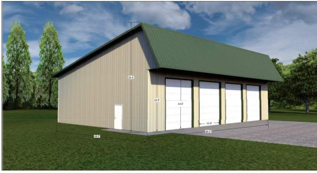
3:12 TO 7:12 ROOF PITCH SHALL BE MEASURED FROM THE GROUND TO A POINT OF THE ROOF VERTICALLY HALFWAY BETWEEN EAVE POINT AND RIDGE
