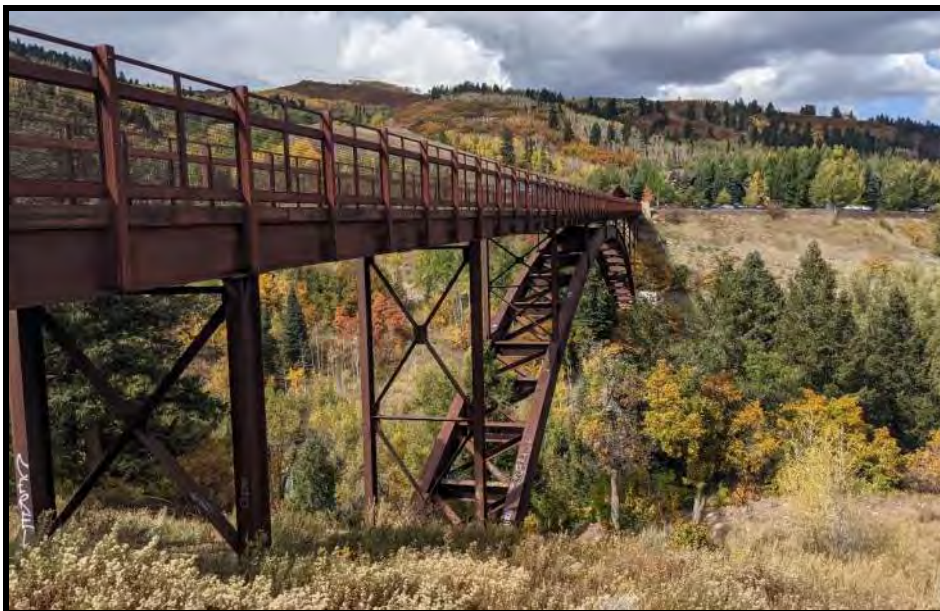
Figure 4-4: Terral Wade Bridge (Tiehack Nordic Bridge, 605 LF) Aspen, Colorado. Weathering Steel Deck Arch
