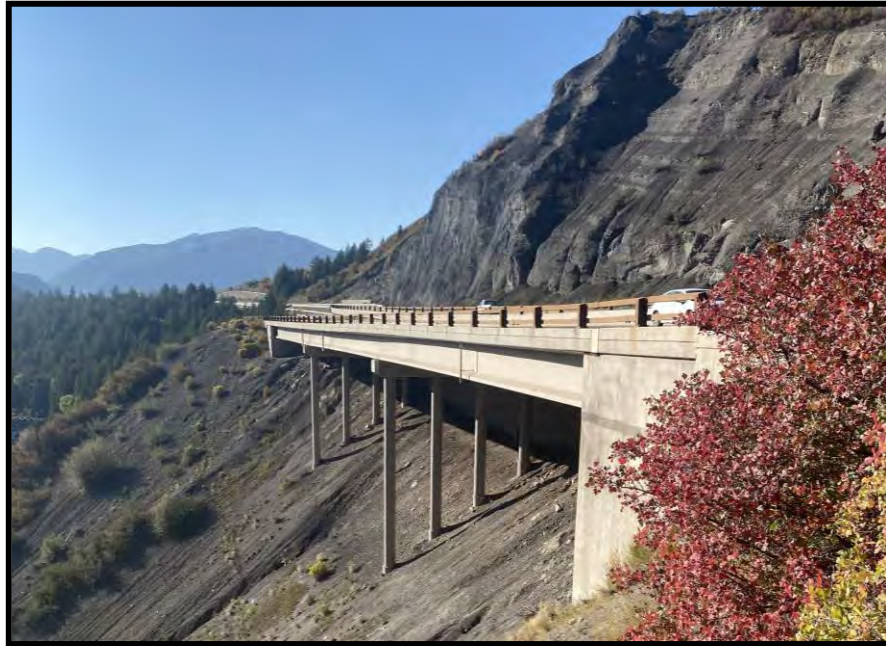
Figure 3-15: Looking South at Existing Shale Bluffs Bridge
