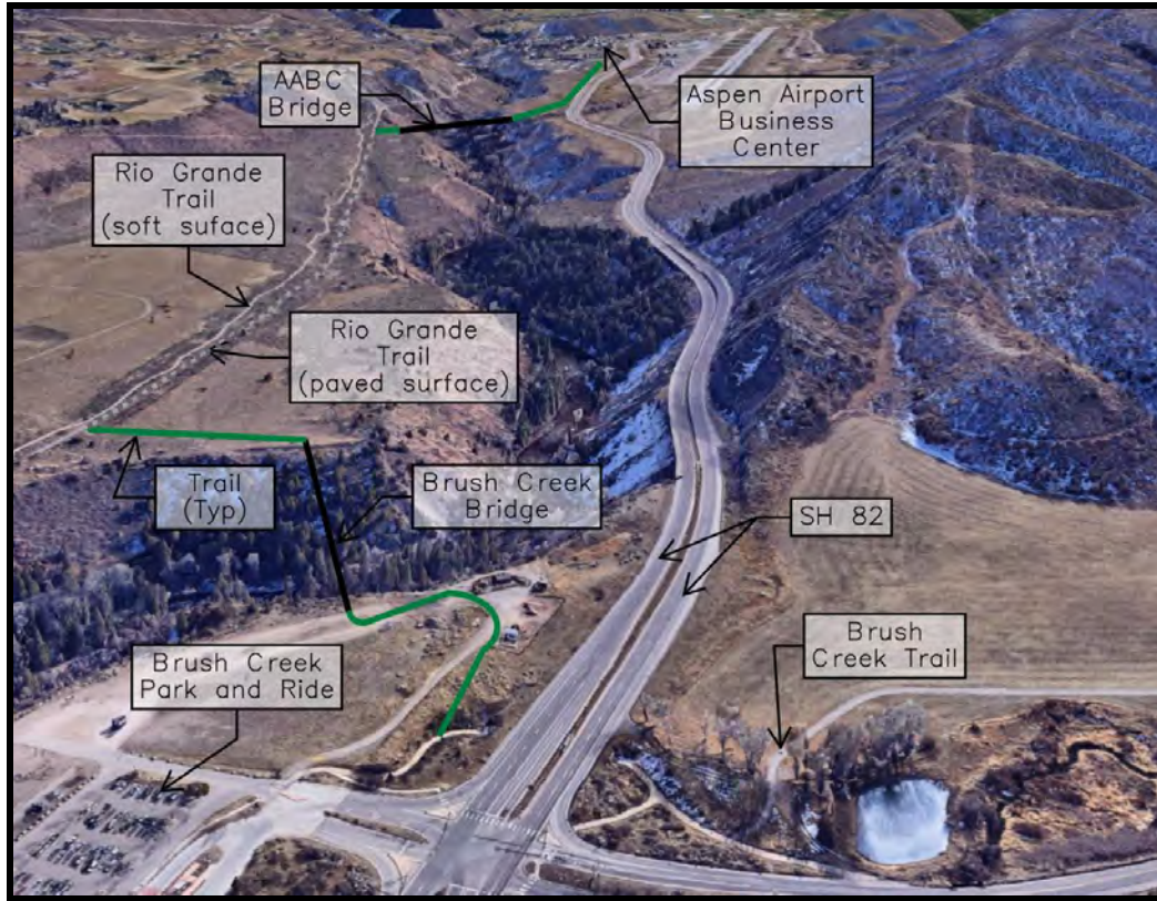
Figure 4-1: Bridge Location Aerial Overview (Imagery Courtesy of Google Earth)
