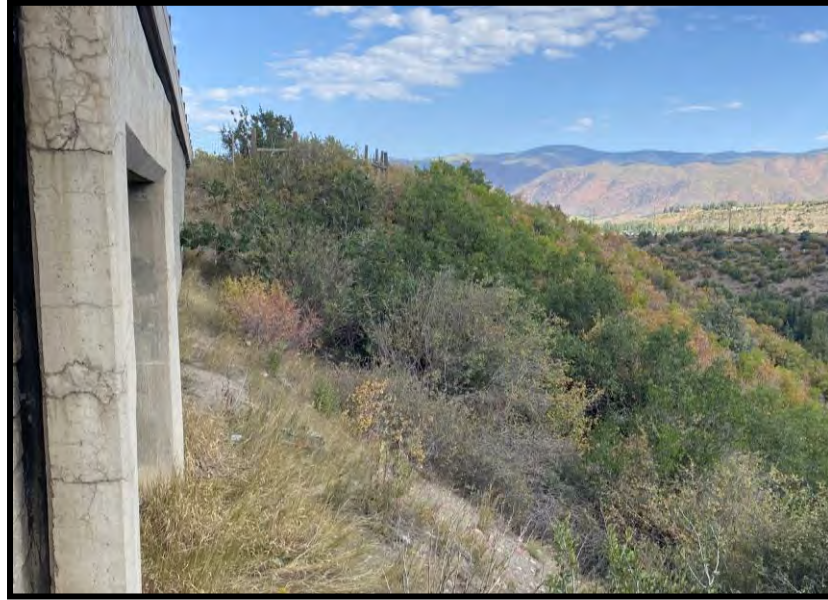
Figure 3-17: Looking North at Existing Box Culvert under SH82
