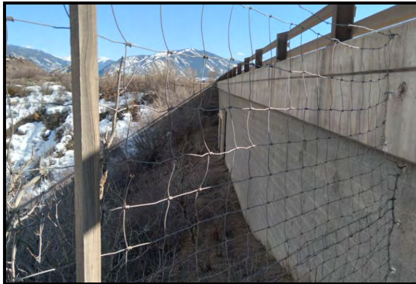
Figure 3-18: Looking South at Existing SH82 Wall and Box Culvert
