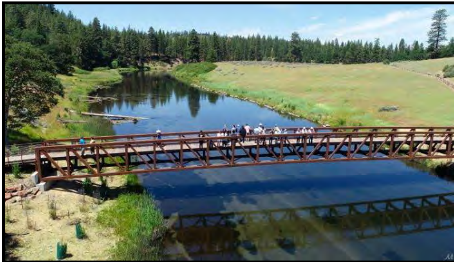
Figure 4-11: Prefabricated Weathering Steel Truss Bridge, Hat Creek, CO (Imagery Courtesy of Excel Bridge) (Note this is a half through truss)
