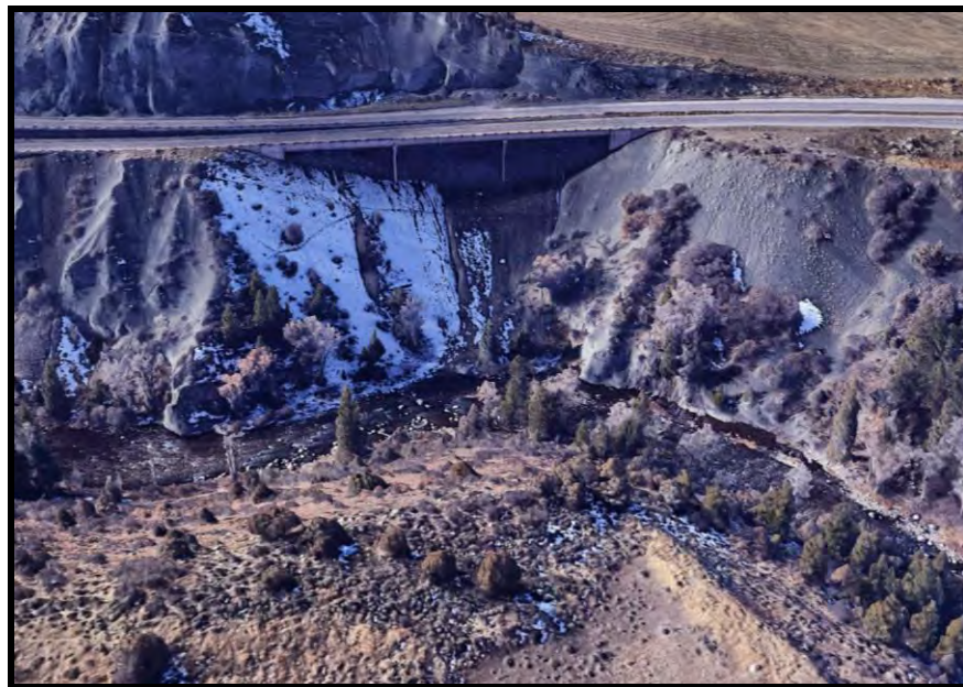
Figure 3-16: Looking West at Shale Bluffs and SH82 Bridge (Imagery Courtesy of Google Earth)
