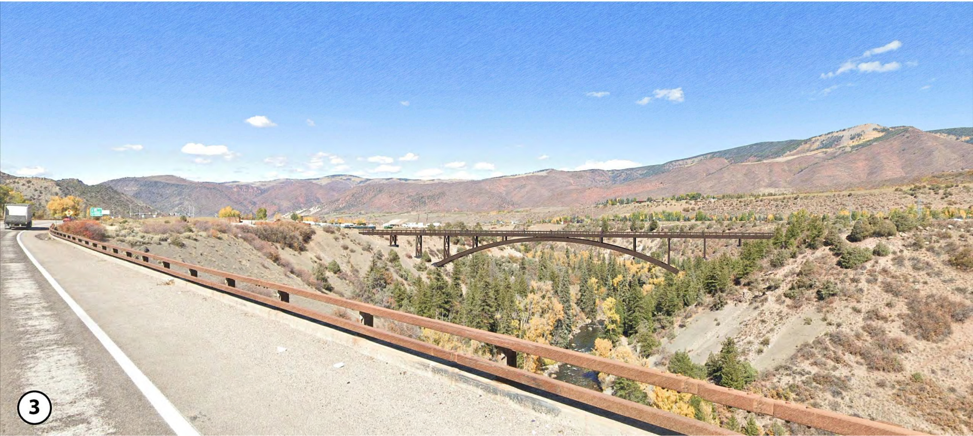
Brush Creek Bridge, Looking Northeast (towards Woody Creek) from SH82
