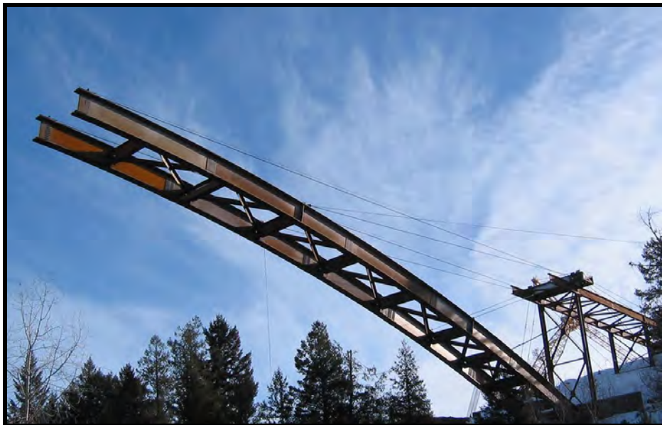
Figure 4-7: Terral Wade Bridge During Construction (Imagery Courtesy of Modjeski and Masters)
