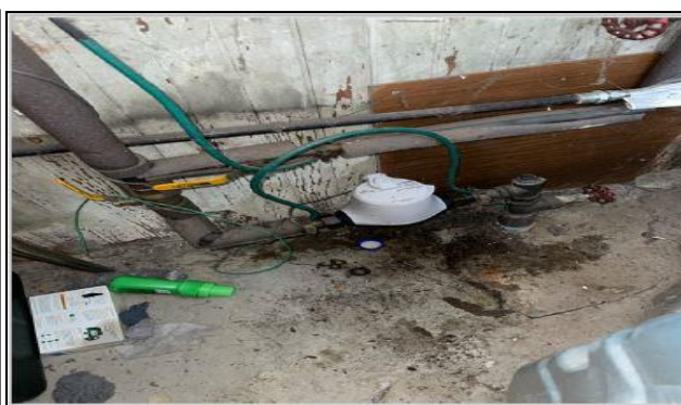
New Meter Install
