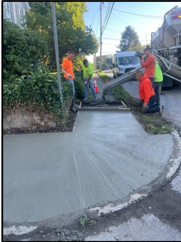
Highway and Water Departments collaborating on the installation of ADA ramps in preparation for milling and paving
