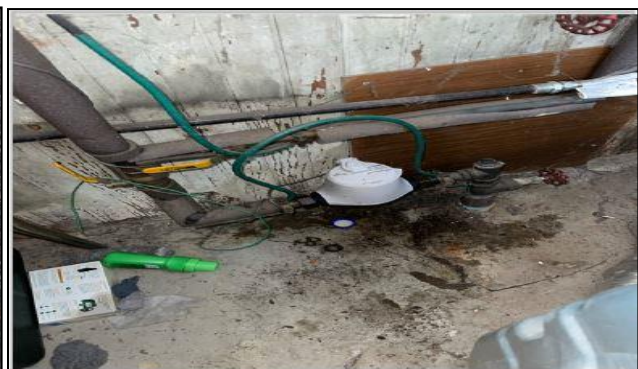
New Meter Install
