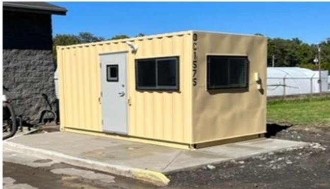
New Hauler Station Office
