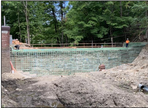
Upstream Pocket Dam Rebar Forming
