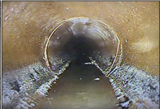
Wesley Ave. Sewer Main
