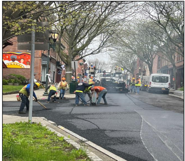
Paving of Main Street
