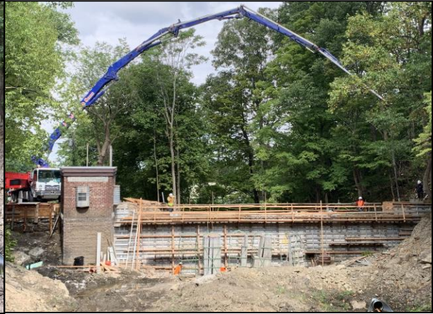
Pumping of Concrete
