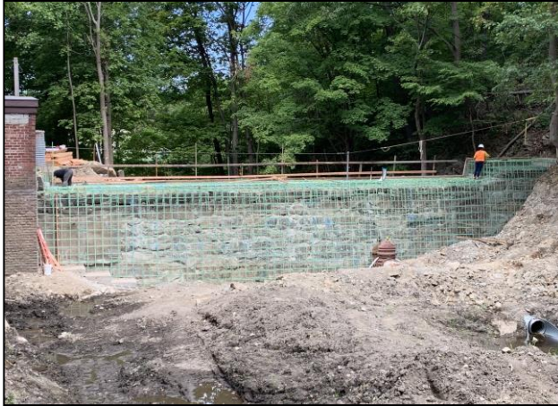
Upstream Pocket Dam Rebar Forming
