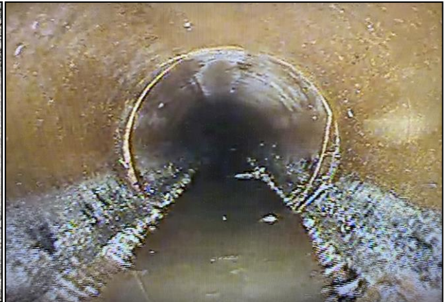
Wesley Ave. Sewer Main
