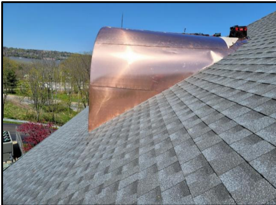
New roof installed at City Hall, including copper wrapped dormers
