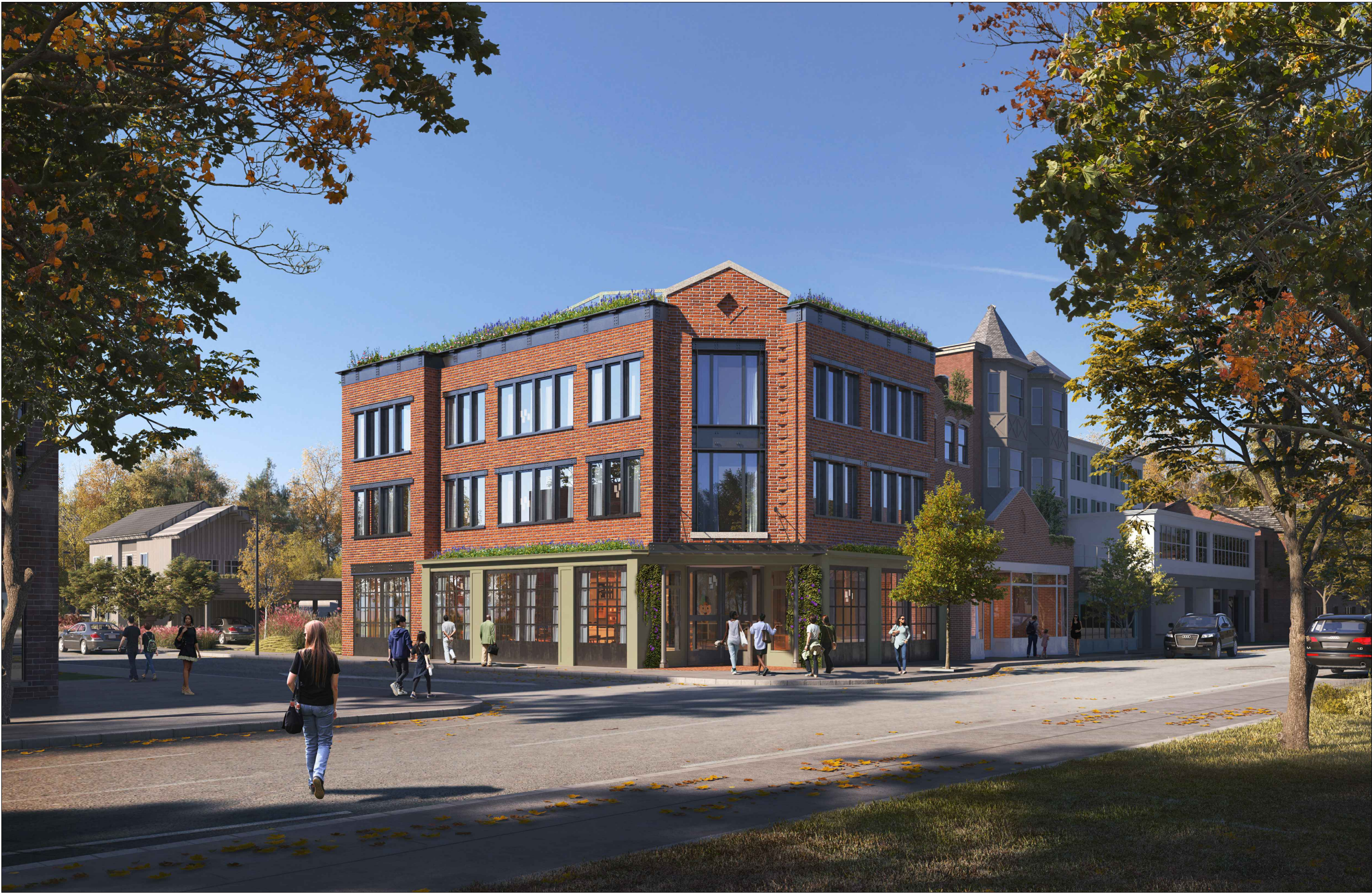
Main Building: View from Corner
