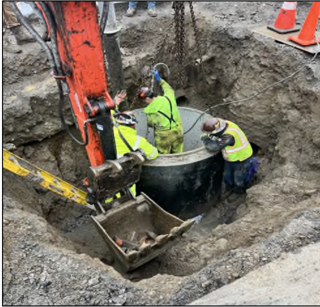
Manhole Replacement- Main St and Teller Ave
