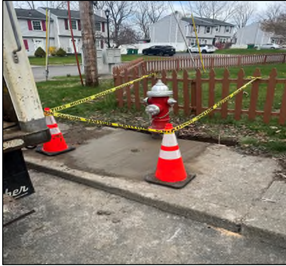
Repaired hydrant valve and sidewalk
