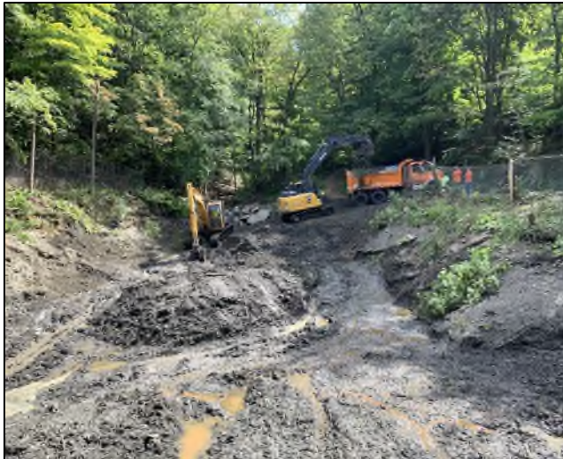
Dredging of Pocket Reservoir
