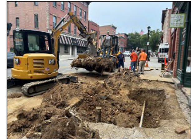
Highway Staff Replacing Main Street Sidewalk & Street Tree
