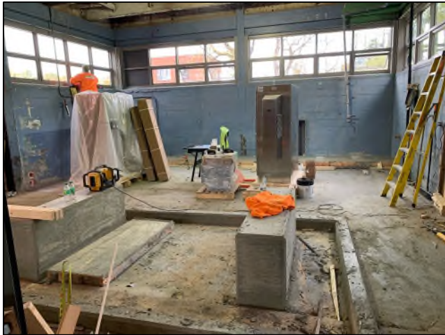
Interior Renovations of Dewatering Bldg.
