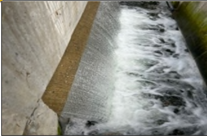
Clean Effluent Discharged to Hudson River
