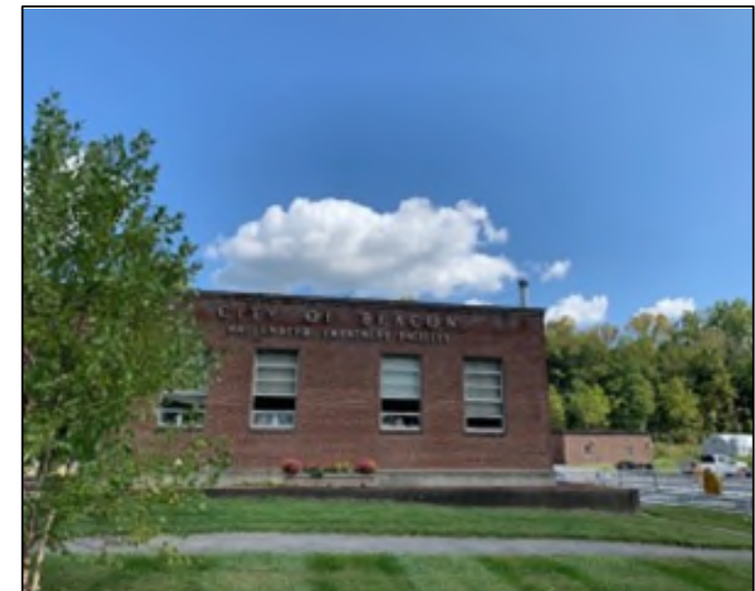
WWTP Administration Building
