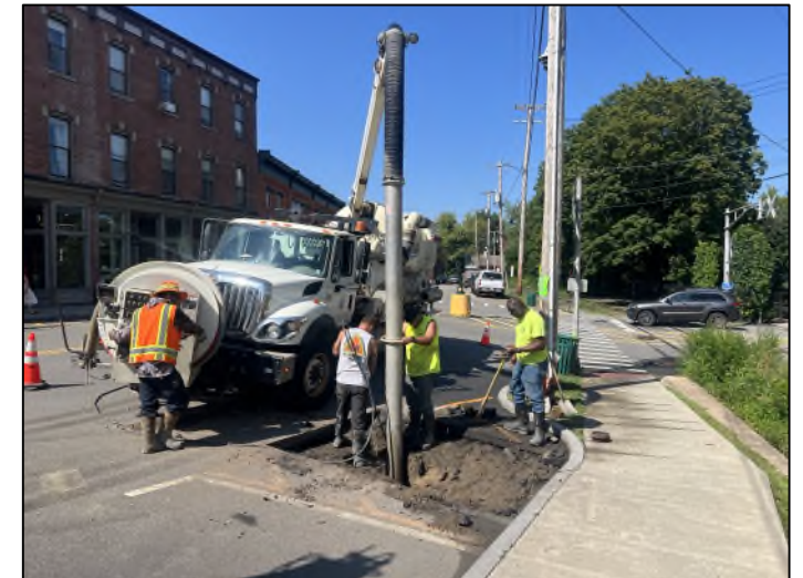
Hydrant Lateral Repair Main St near Dummy Light
