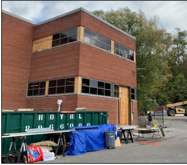
Solids Dewatering Project Started Early 2025
