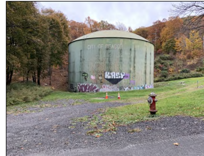
Mount Beacon Water Storage Tank
