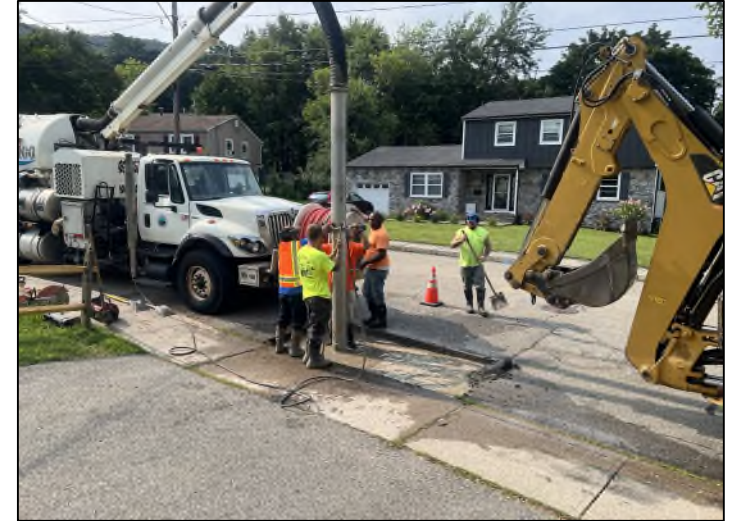
Water main repair on Heaney Drive
