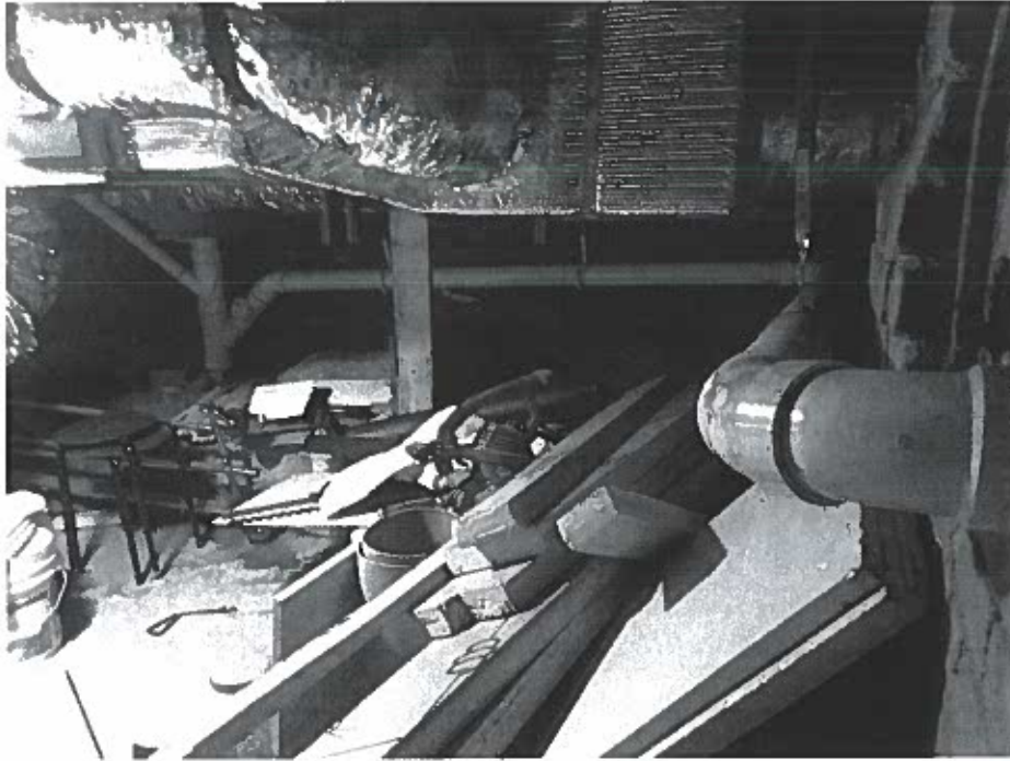
View of the sewer lines as they lead to the raw invert outlet.
