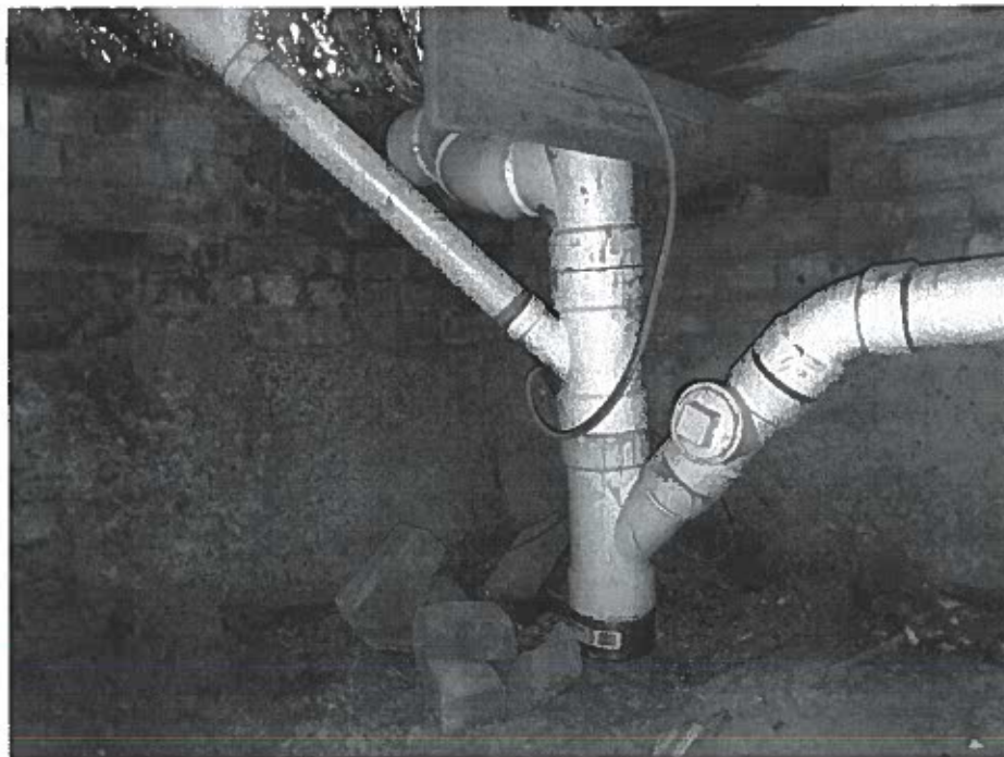
View of the raw invert outlet connection near the basement's southeastern corner.
