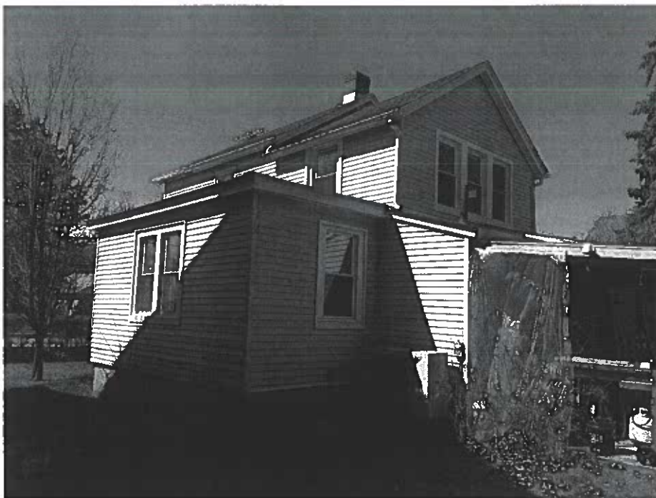
View of the second-floor gutters along the residence's south side as seen from southeast of the building.
