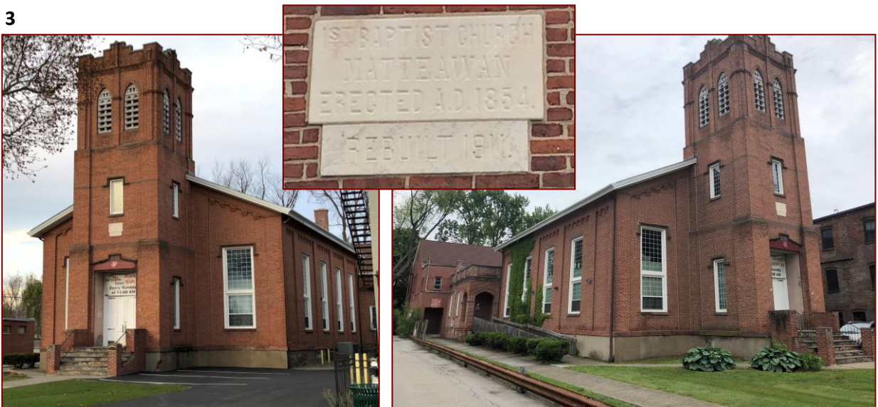
372 Main Street Front View and East Side
