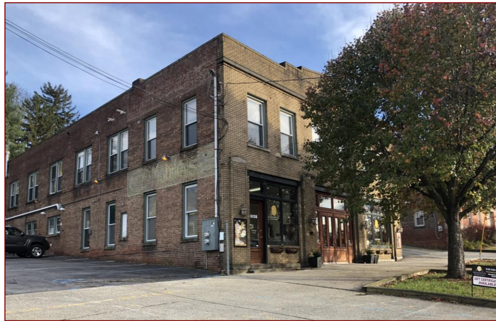
Front View from North
