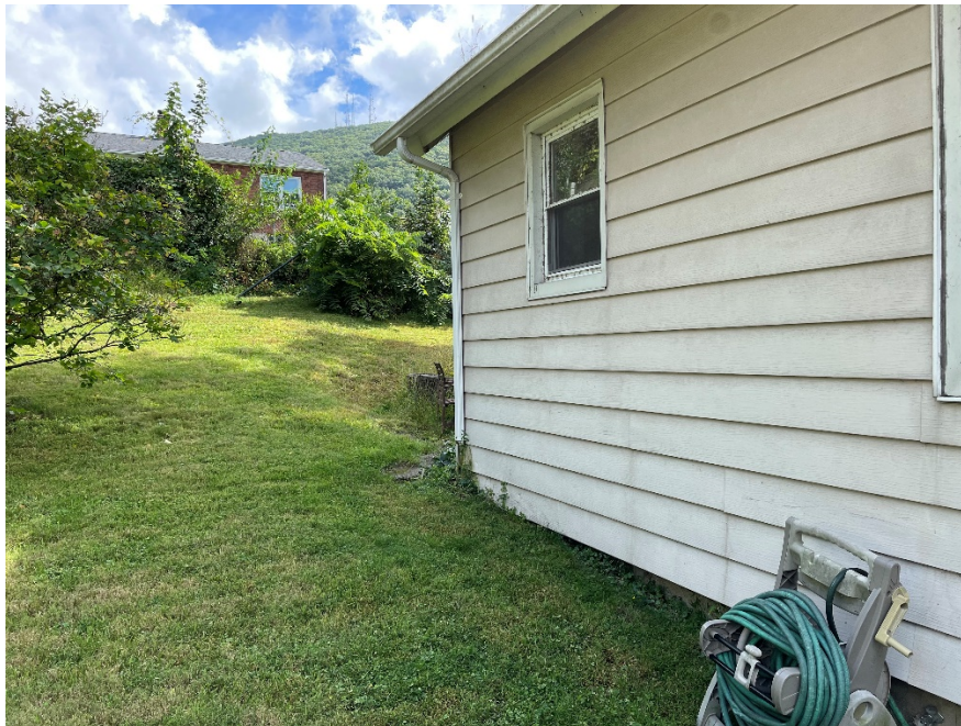
Figure 1- Roof Leader Southeast Corner
