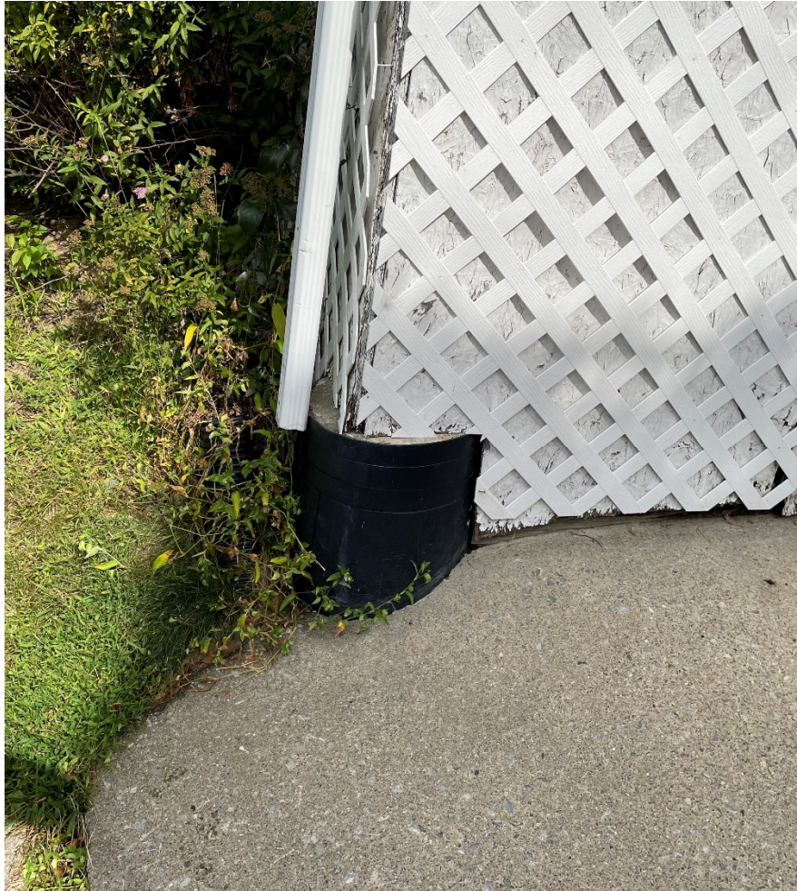
Figure 2- Roof Leader Northwest Corner
