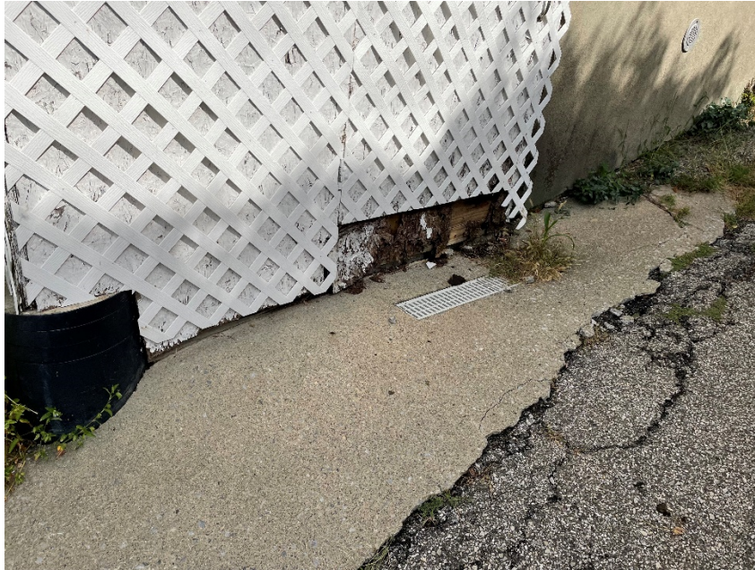
Figure 3- Trench Drain at Basement Entrance
