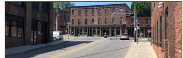
East Main Street is overly wide with no street trees or landscaped buffer for pedestrians from passing traffic.
