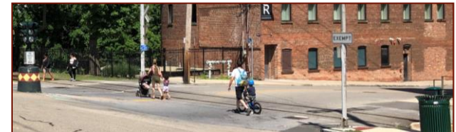
The East Main Street crossing has no crosswalk and remaining rail tracks that can act as a trip hazard.
