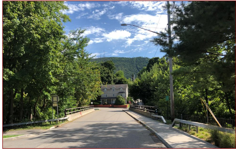
View East across Bridge
