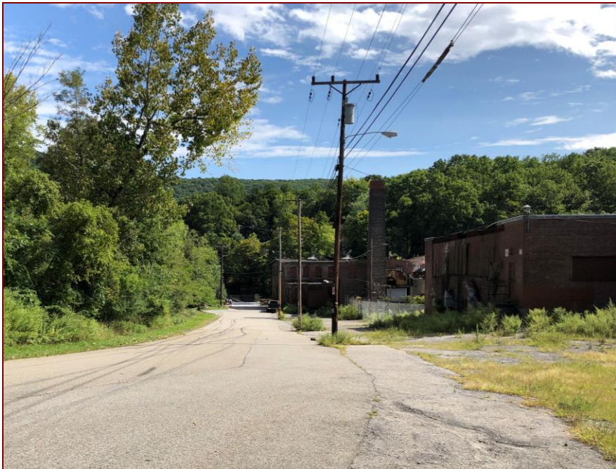
View toward the Bridge from the Tunnel
