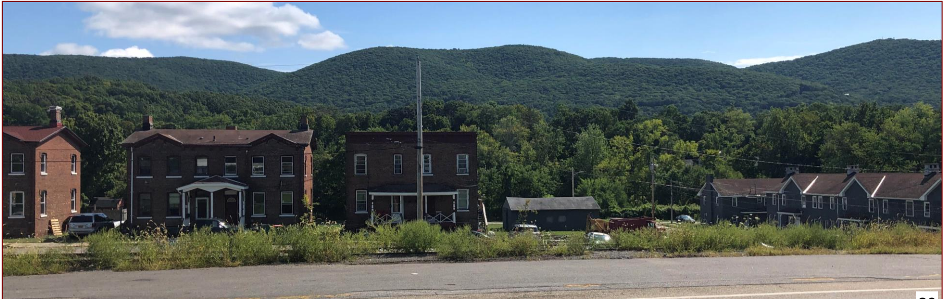
Route 52 at State Street
