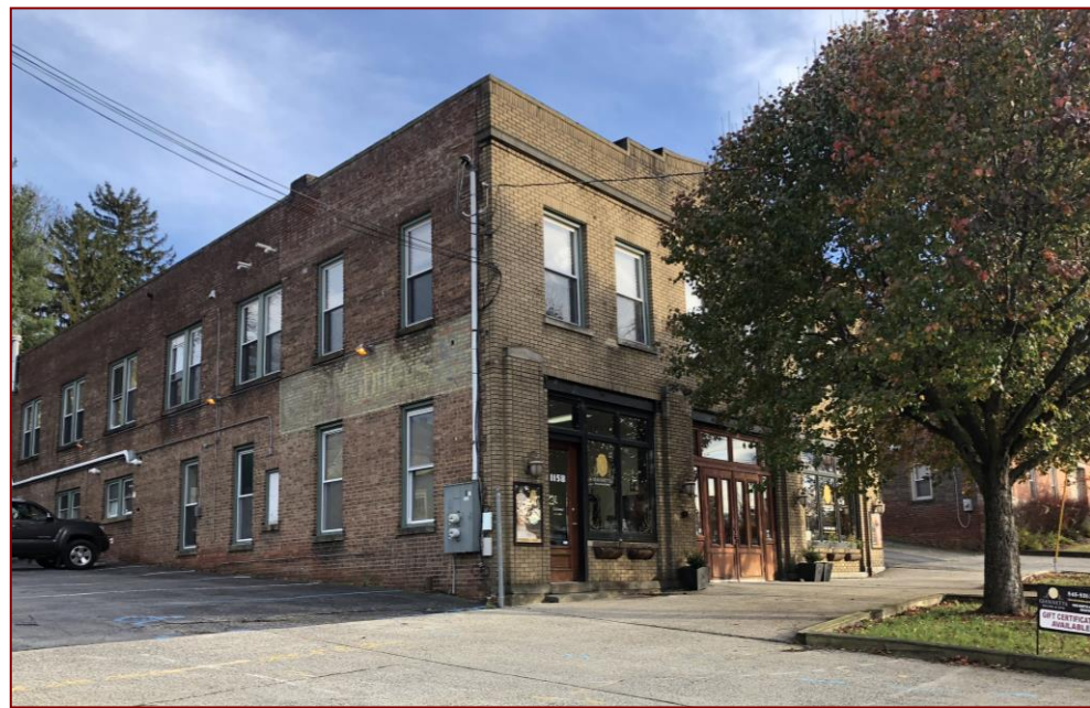
Front View from North
