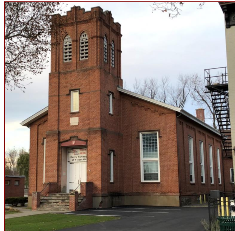
Front View and East Side
