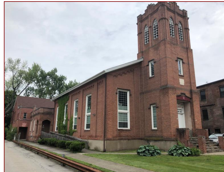
Front View and West Side
