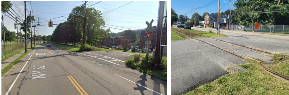
Figure 7. At Grade Rail Crossing at Mill Street (Left: From Fishkill Ave.; Right: From Mill St.)
