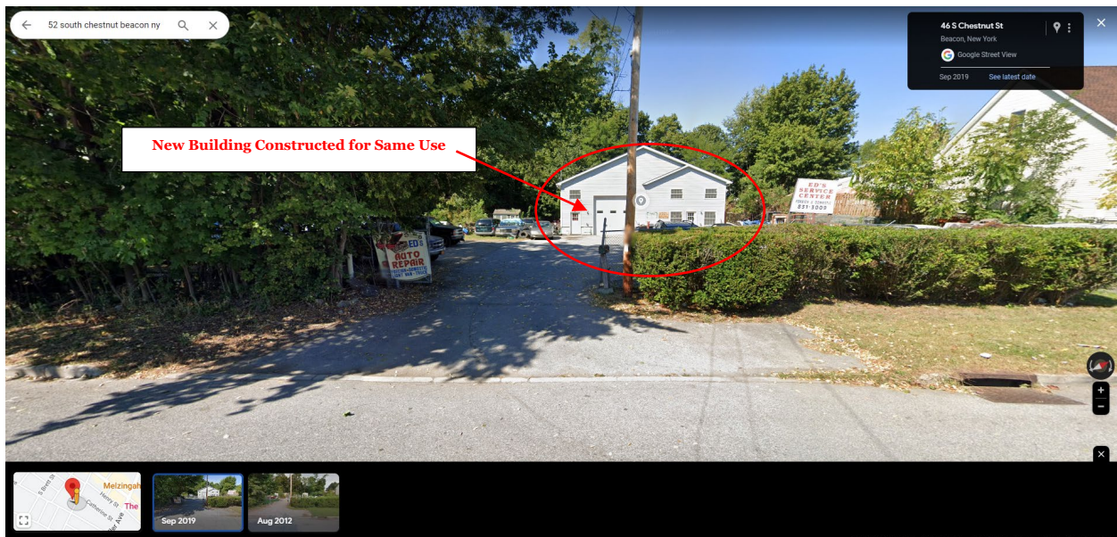
2019 Google Streetview Showing South Chestnut Property After New Autobody Building was Constructed Several Years After Being Destroyed by Snowstorm
