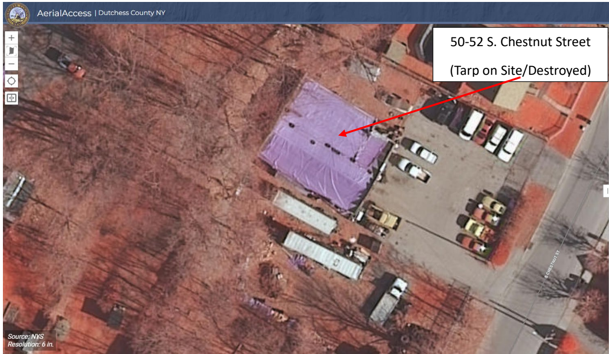
2009 Dutchess County GIS Aerial of 50-52 South Chestnut Street
