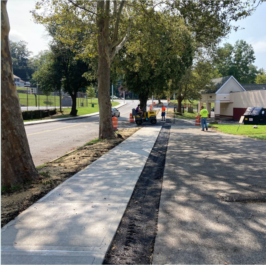
South Avenue Sidewalk Replacement (2023) Funded by Community Dev. Block Grant Funds
