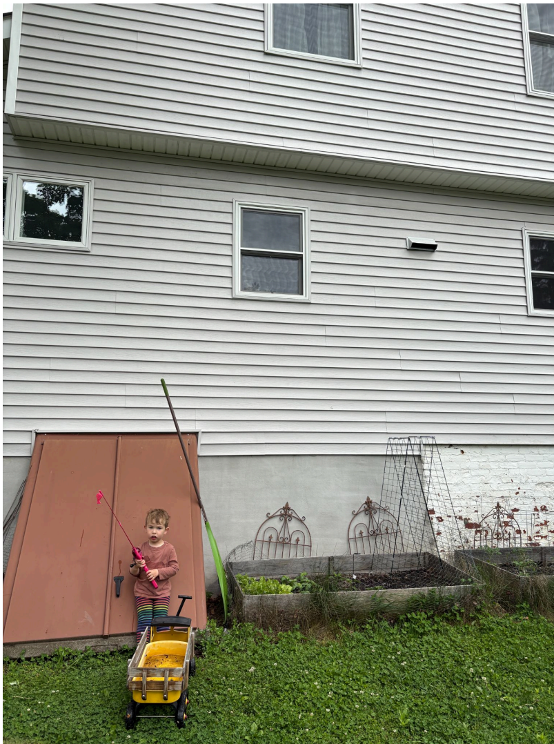
Rear of house seen from outside. The area directly behind the house has critical basement access and an existing garden.
