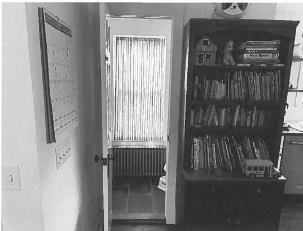
Area of proposed downstairs addition seen from inside. The existing bathroom seen here would be condensed so this doorway could lead to the new downstairs office.
