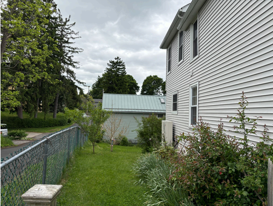
Area of proposed addition seen from outside, facing south. 7 Odell Street can be seen in the background.
