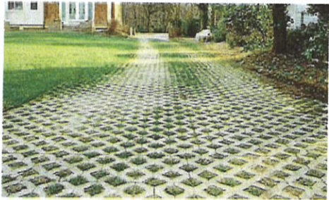
PAVER STYLE FOR DRIVEWAY ALREADY INSTALLED AS PATIO BUT BUILT FOR DRIVEWAY
