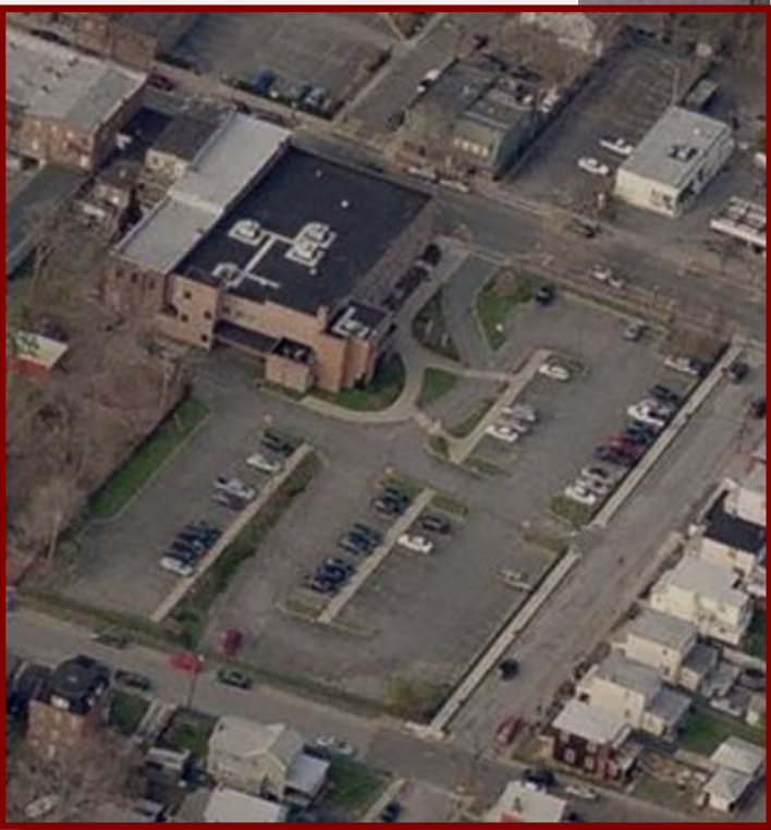
Existing 92-Space Lot
