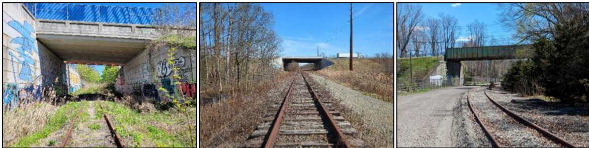
Figure 15: Overpass Structures 1 (Left), 2 (Center), and 3 (Right).
