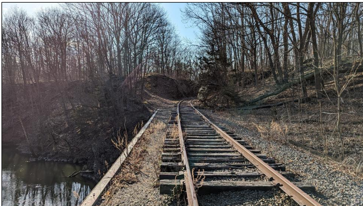
Figure 12: Bridge 3 - Town of Fishkill Looking West
