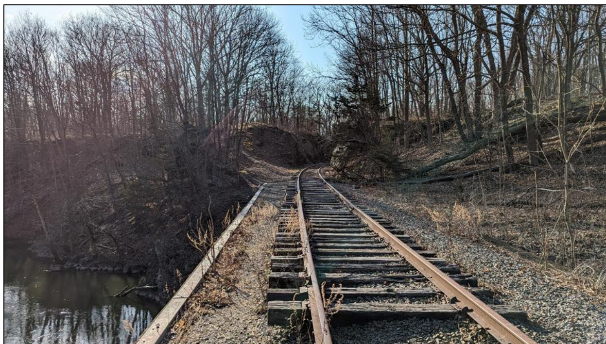
Figure 12: Bridge 3 - Town of Fishkill Looking West
