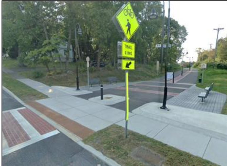
Figure 29: Northside Line Trail Entrance with signage, lighting, benches, regulatory, and informational signage.
