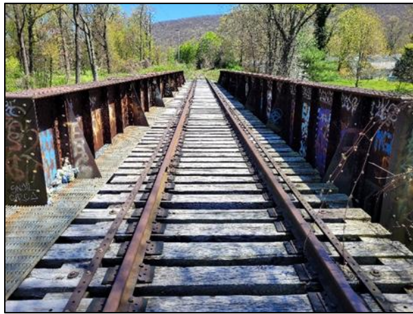
Figure 7: Existing three-span structure with through-girder section.
