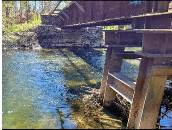
Figure 8: Existing two-span bridge with steel pier and stone masonry foundations.
