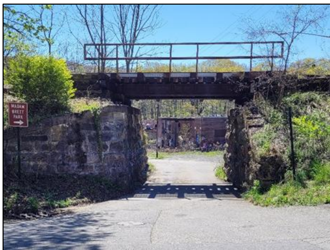
Figure 5: Stone masonry bridge with steel girders.
