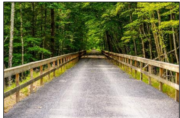
Figure 2: Example of Safety Railing
