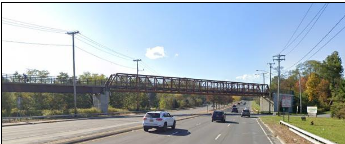
Figure 20: Example of a rail trail bridge – WRS Dutchess Rail Trail over State Route 55.
