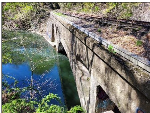
Figure 6: Existing concrete arch bridge.
