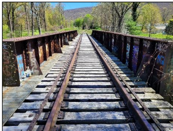
Figure 7: Existing three-span structure with through-girder section.
