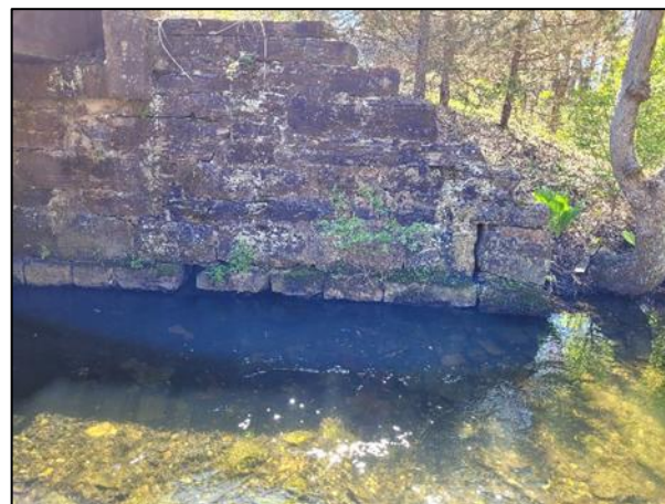
Figure 9: Stone masonry foundation as seen on Bridge 6.
