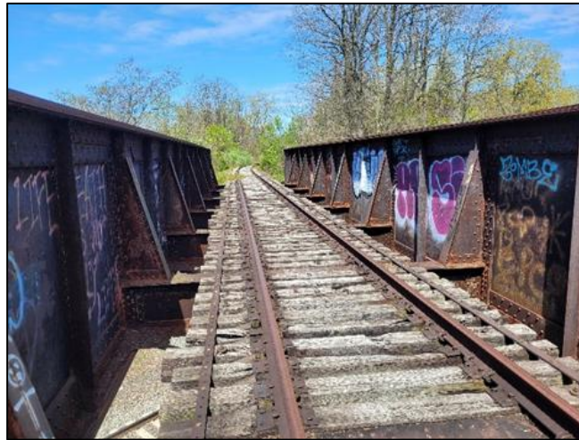
Figure 4: Existing through-girder structure over Metro-North Hudson Line.
