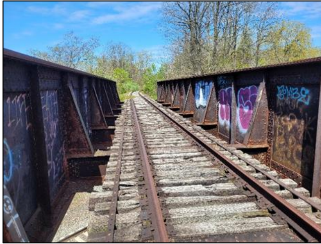
Figure 4: Existing through-girder structure over Metro-North Hudson Line.
