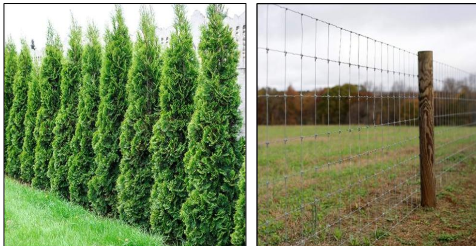
Figure 30: Examples of trail screening: vegetative buffer with evergreen trees (left) and 4-ft high box wire fencing (right).
