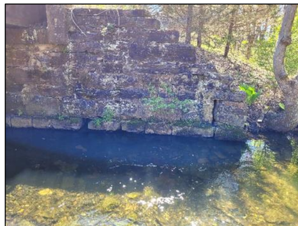
Figure 9: Stone masonry foundation as seen on Bridge 6.
