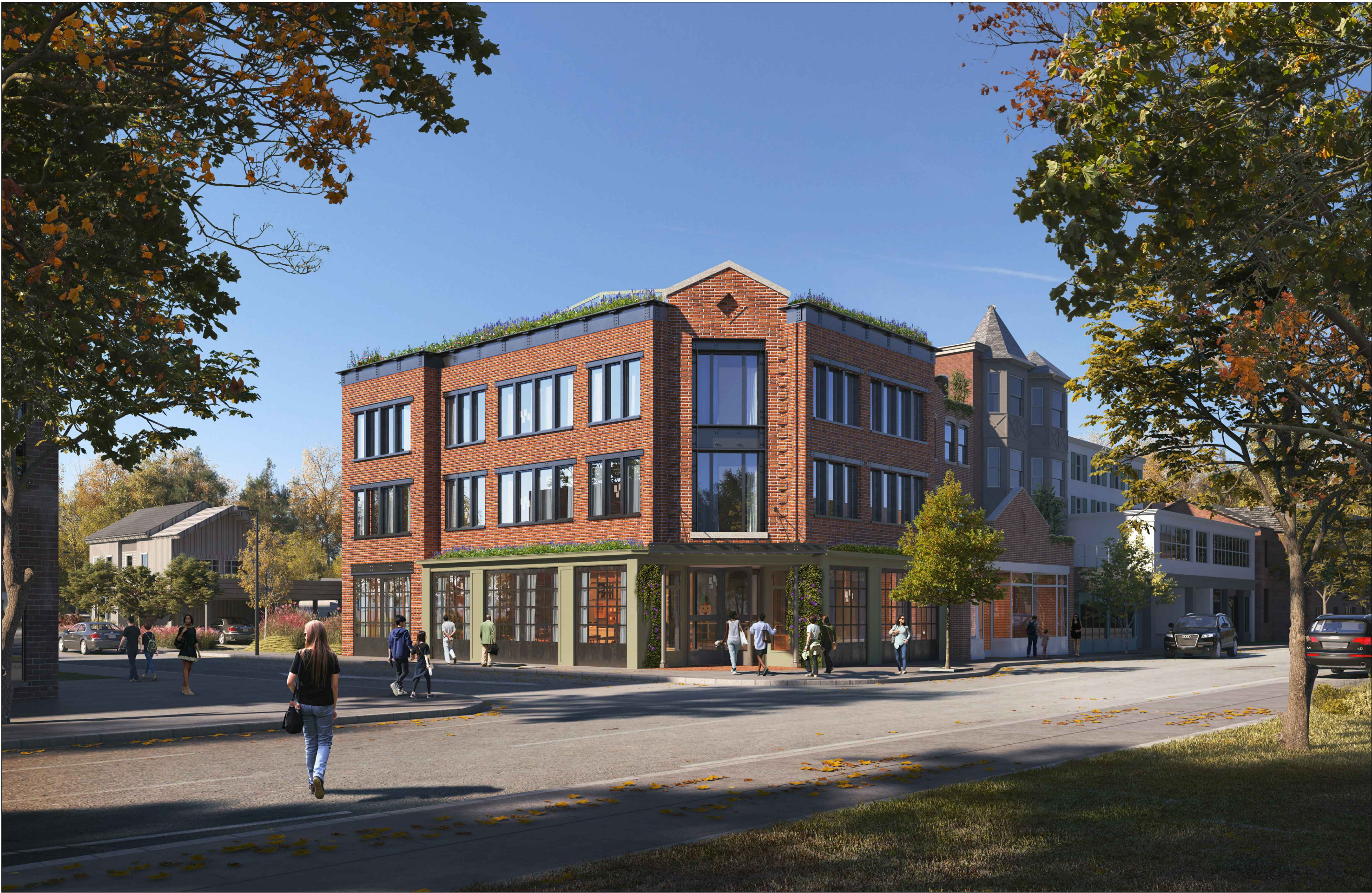
View from Corner
