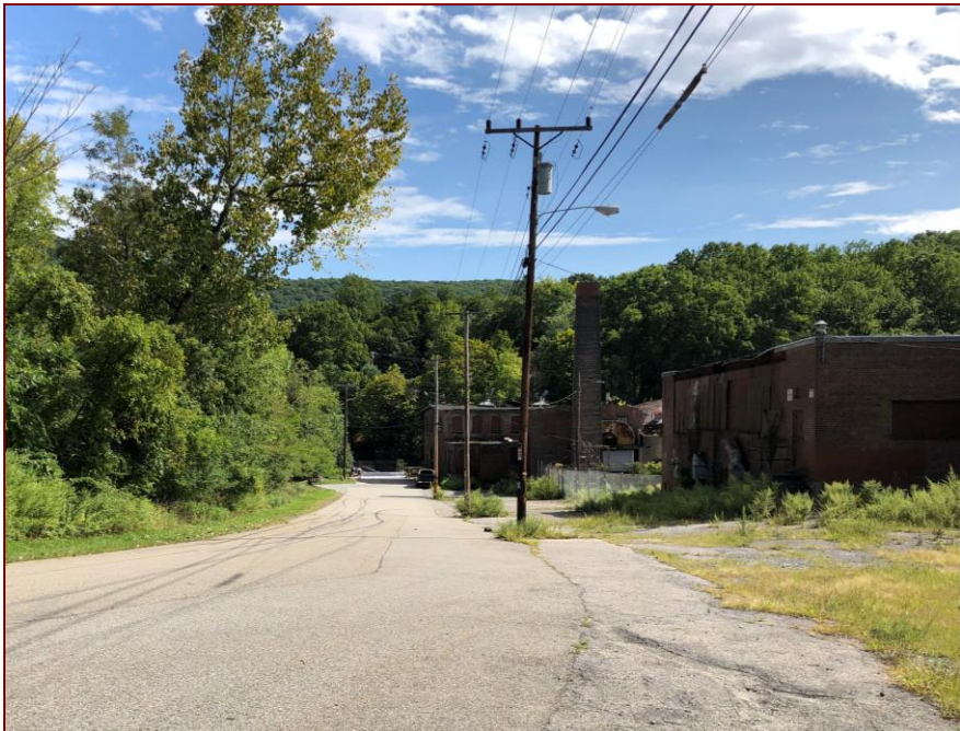
View toward the Bridge from the Tunnel
