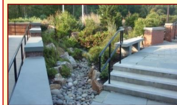
Rain garden built into a planter box at the building entrance.
