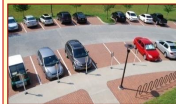
Permeable pavement and brick pavers in the parking lot with reinforced grass overflow parking to the rear.
