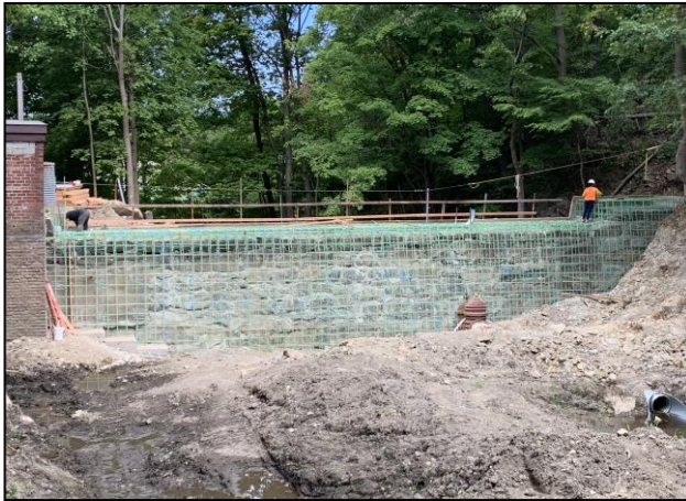
Upstream Pocket Dam Rebar Forming
