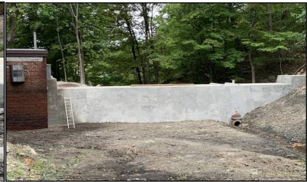
Buttress Removal & Surface Preparation
