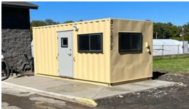
New Hauler Station Office
