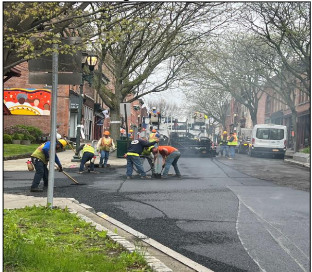
Paving of Main Street
