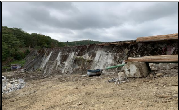
Buttress Removal & Surface Preparation
