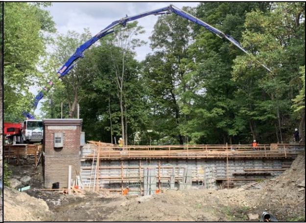
Pumping of Concrete
