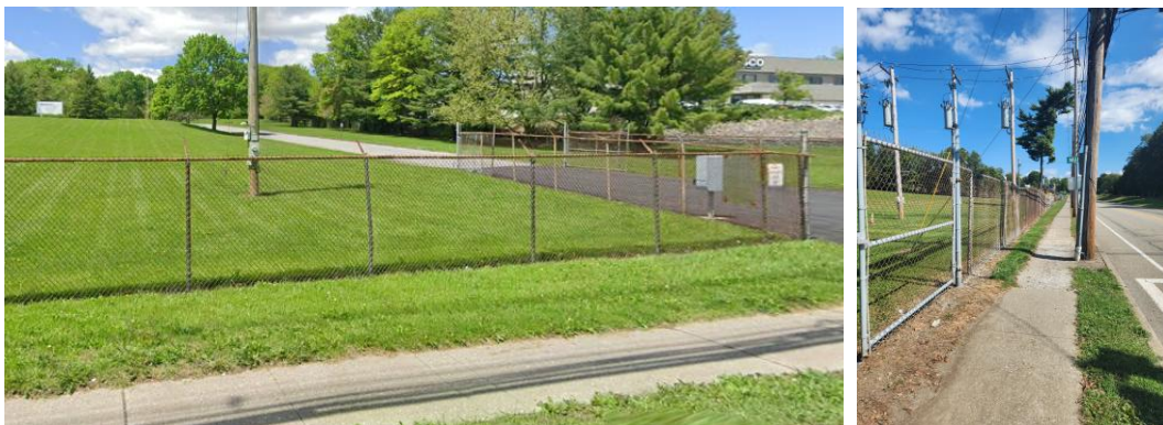
Figure 4. Industrial site boundaries that could benefit from improved landscaping and fencing
