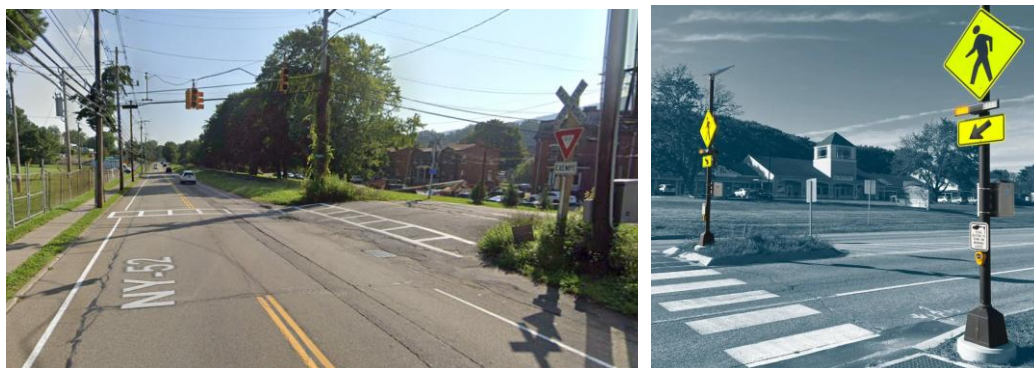
Figure 8. (Left) Existing Intersection at Mill Street (Right) Example of RRFB
