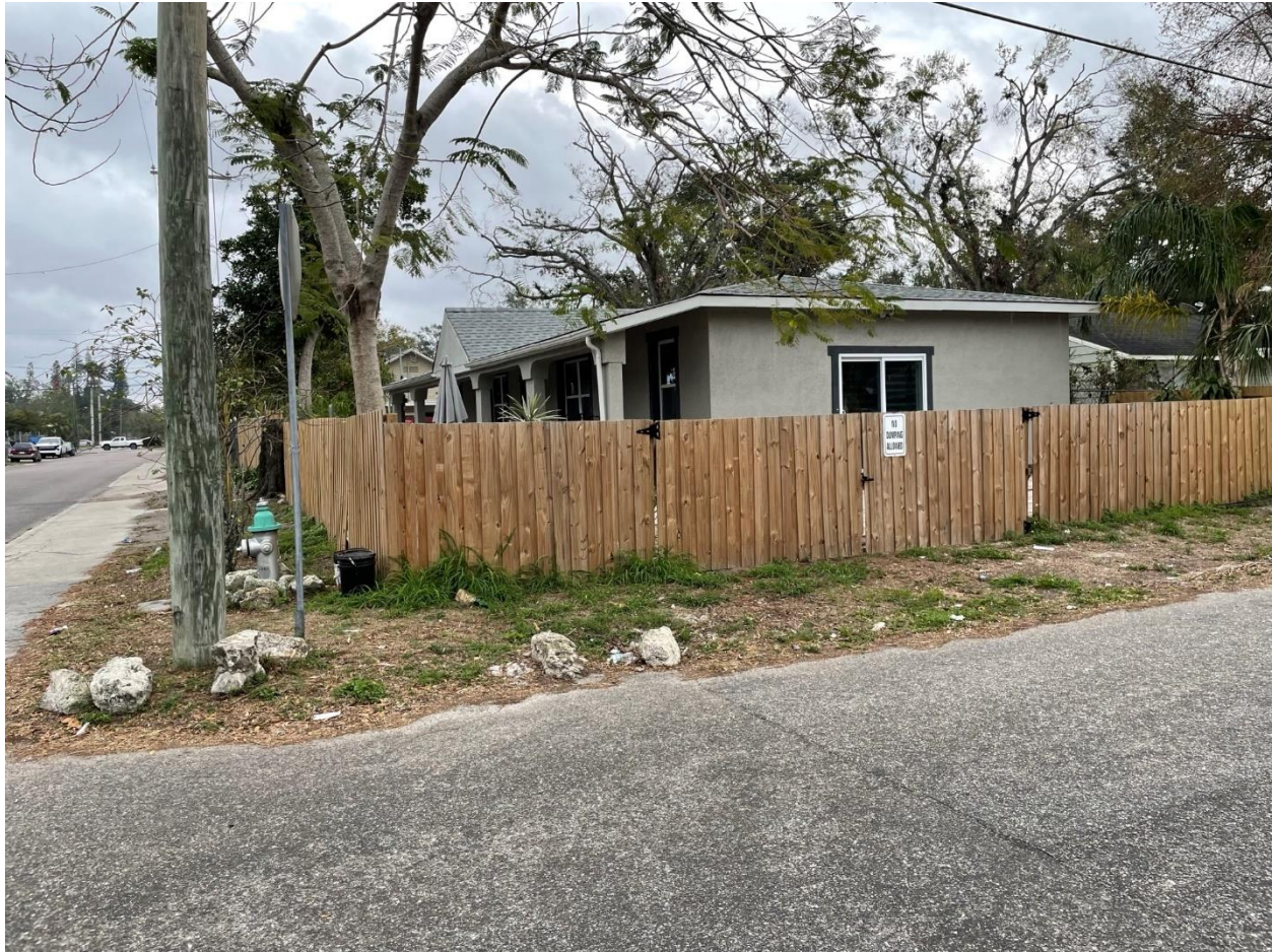
View from 11 th Street West
