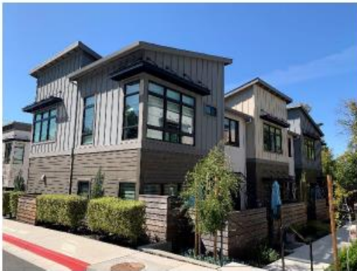
Varied roof forms with change in direction of roof slope, facade projections, and large bay windows.
