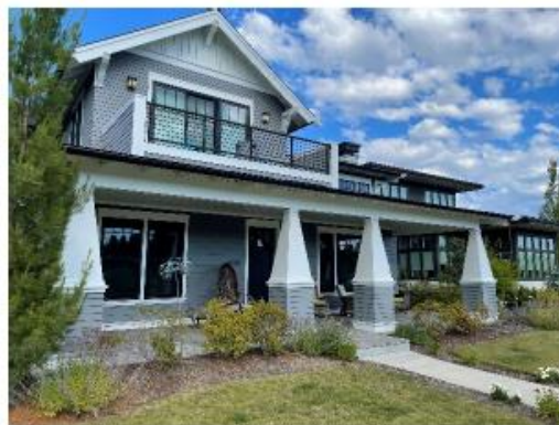
Balcony and covered front porch entry.
