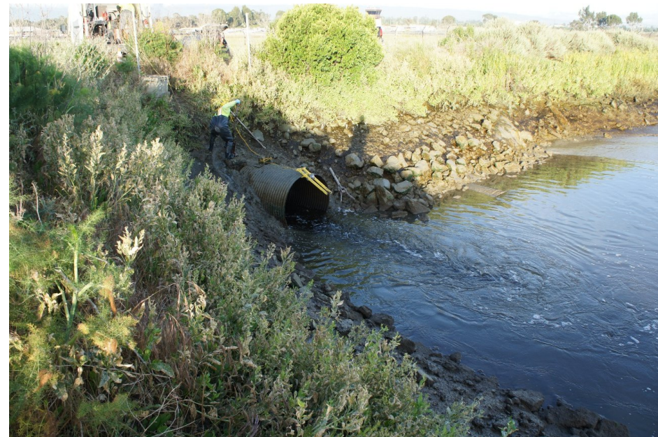
Image from Outfall CCTV inspection
