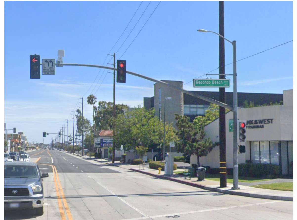
(New traffic signal pole with lighting fixture installed)
