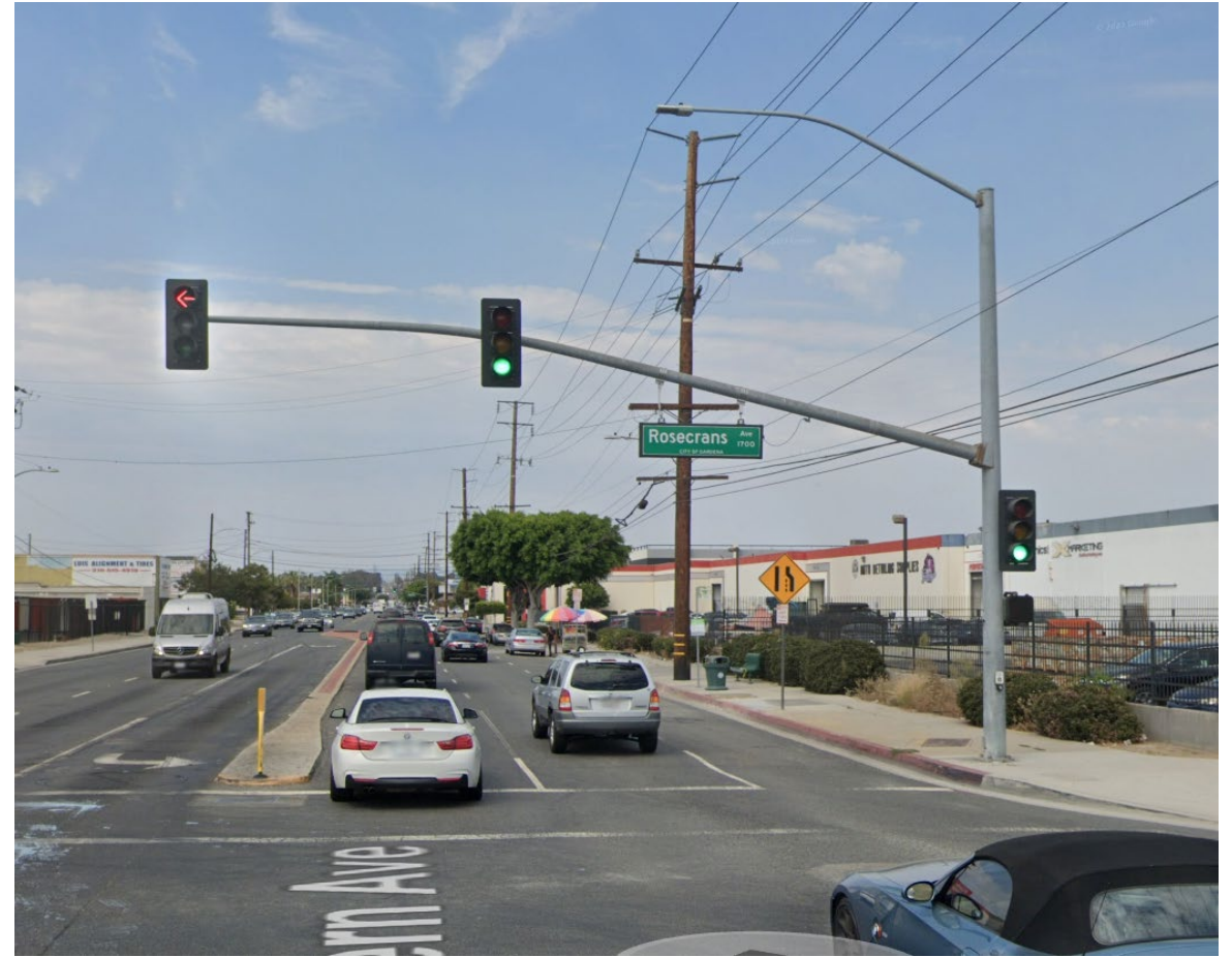
(New traffic signal pole with lighting fixture installed)
