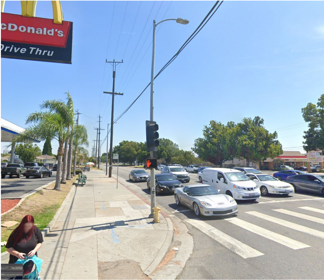
(Existing streetlight with traffic and pedestrian head.)
