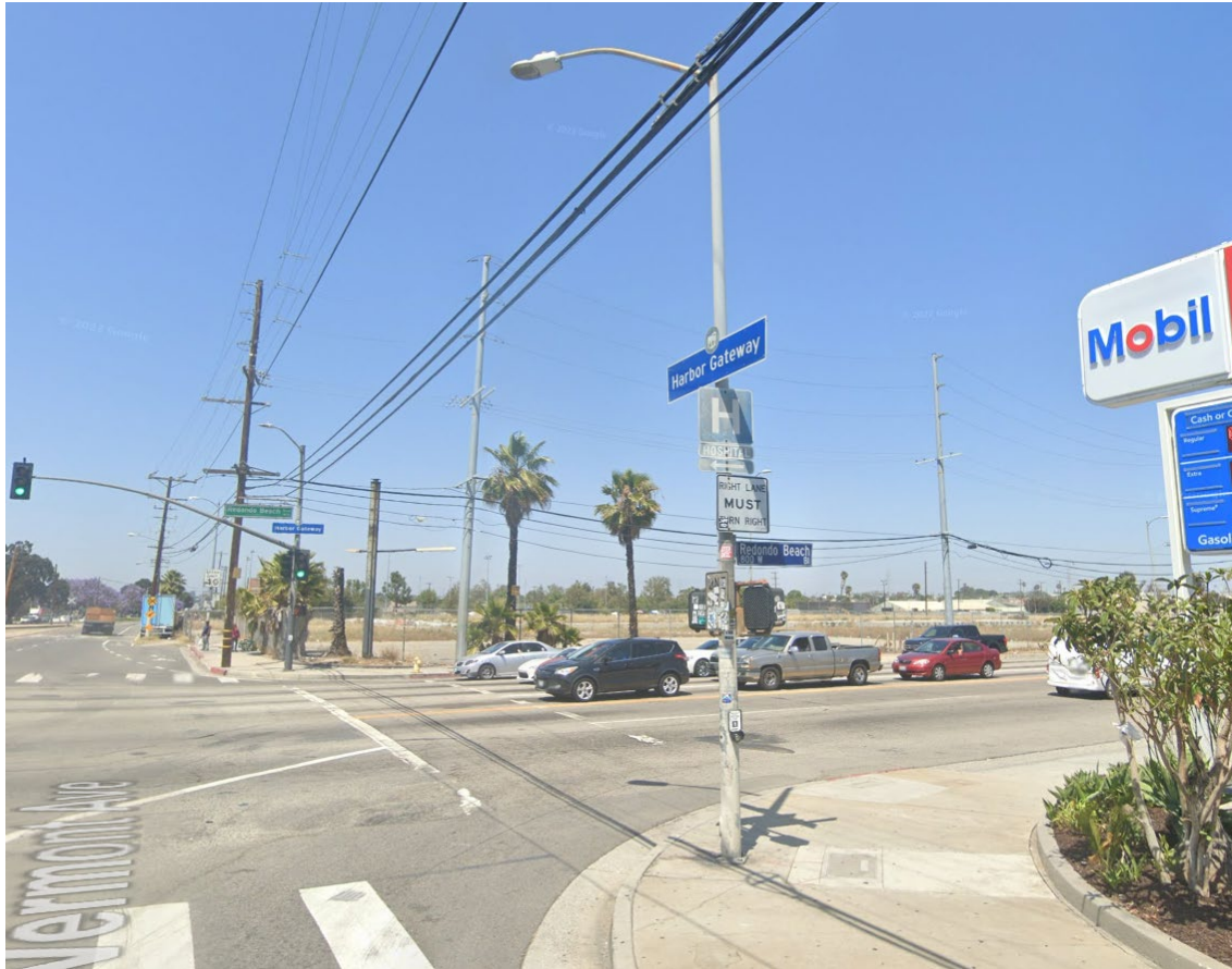
(Existing streetlight with traffic and pedestrian head.)
