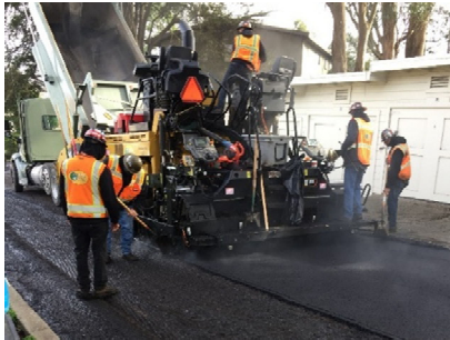
Mill & AC Overlay
