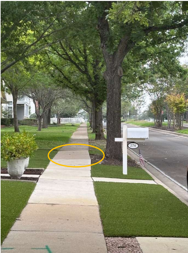
Tree roots causing sidewalk panel displacement, creating an uneven surface
