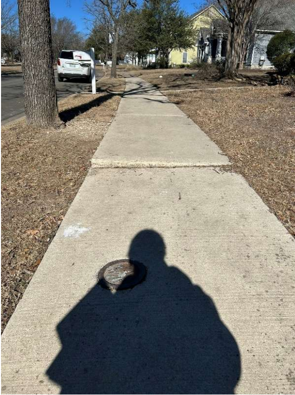
Wastewater cleanout lids located within sidewalk
