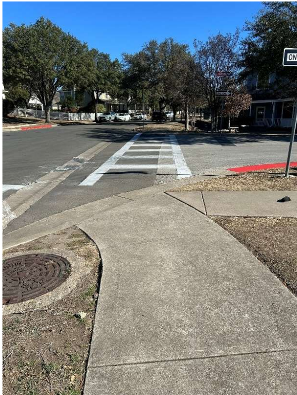
Curb cut ramp does not align with crosswalk and lacks tactile surface to aid vision-impaired pedestrians.
