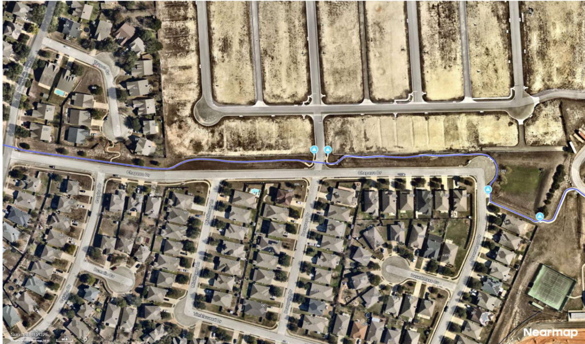
Figure 17 View of locations where concerns were identified along Chaparro Dr
