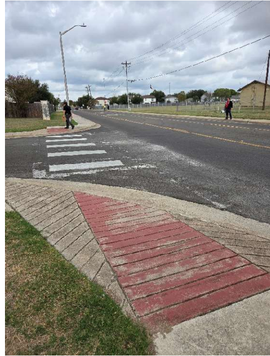
Outdated style of detectable warning surface indicators
