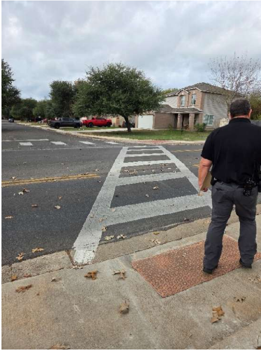
Outdated style of detectable warning surface indicators
