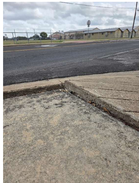
Deficient, uneven sidewalk sections
