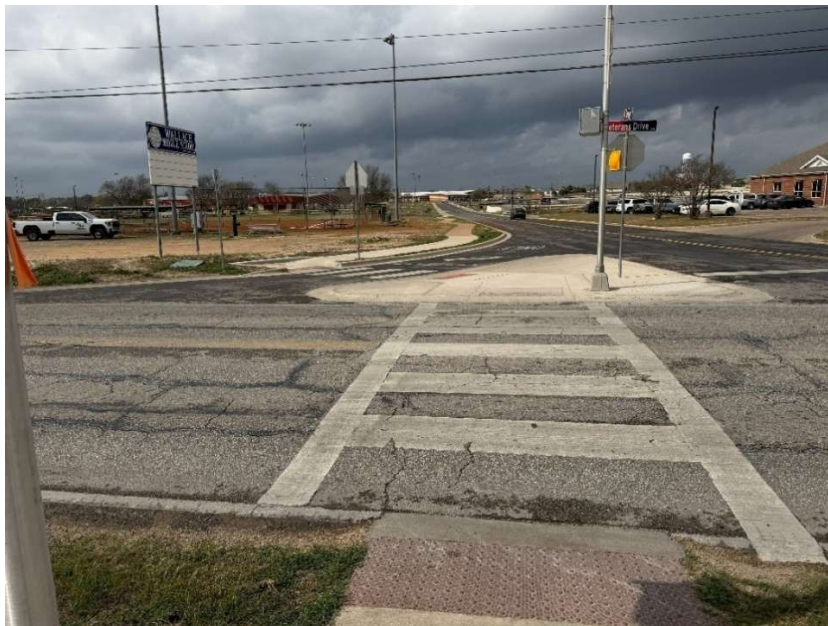
Pedestrian beacon at crosswalk on Veterans Drive is not push-button activated and only operates during school zone hours. Crossing guard is present during school zone hours to alert drivers when pedestrians are crossing the roadway.
