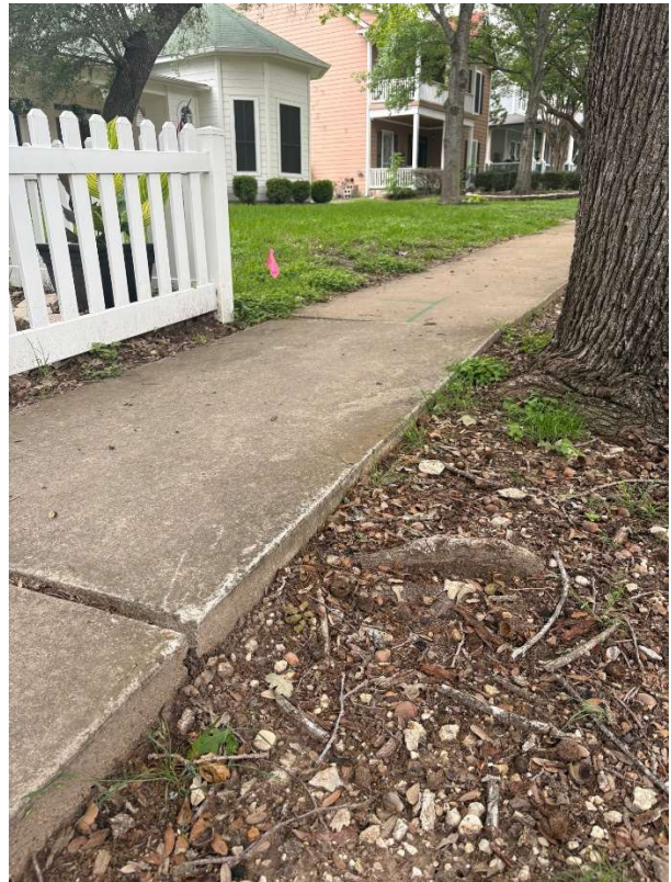
Tree roots causing sidewalk panel displacement, creating an uneven surface
