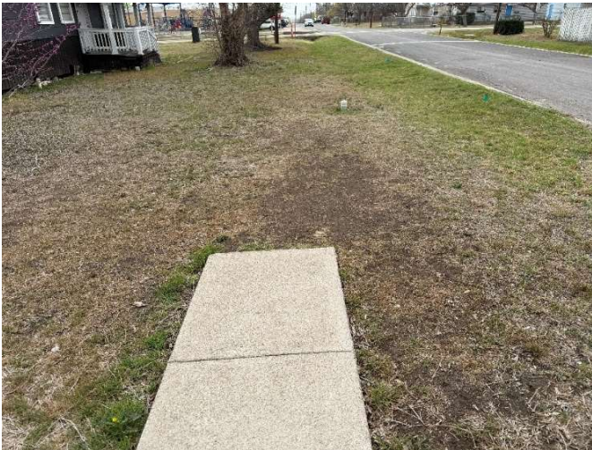
Sidewalk ends before intersection of Blanco Street and N Meyer Street.
