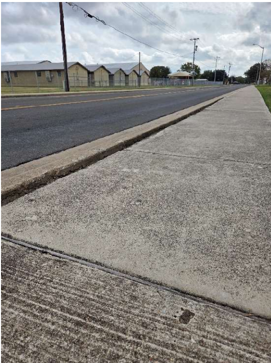
Deficient, uneven sidewalk sections
