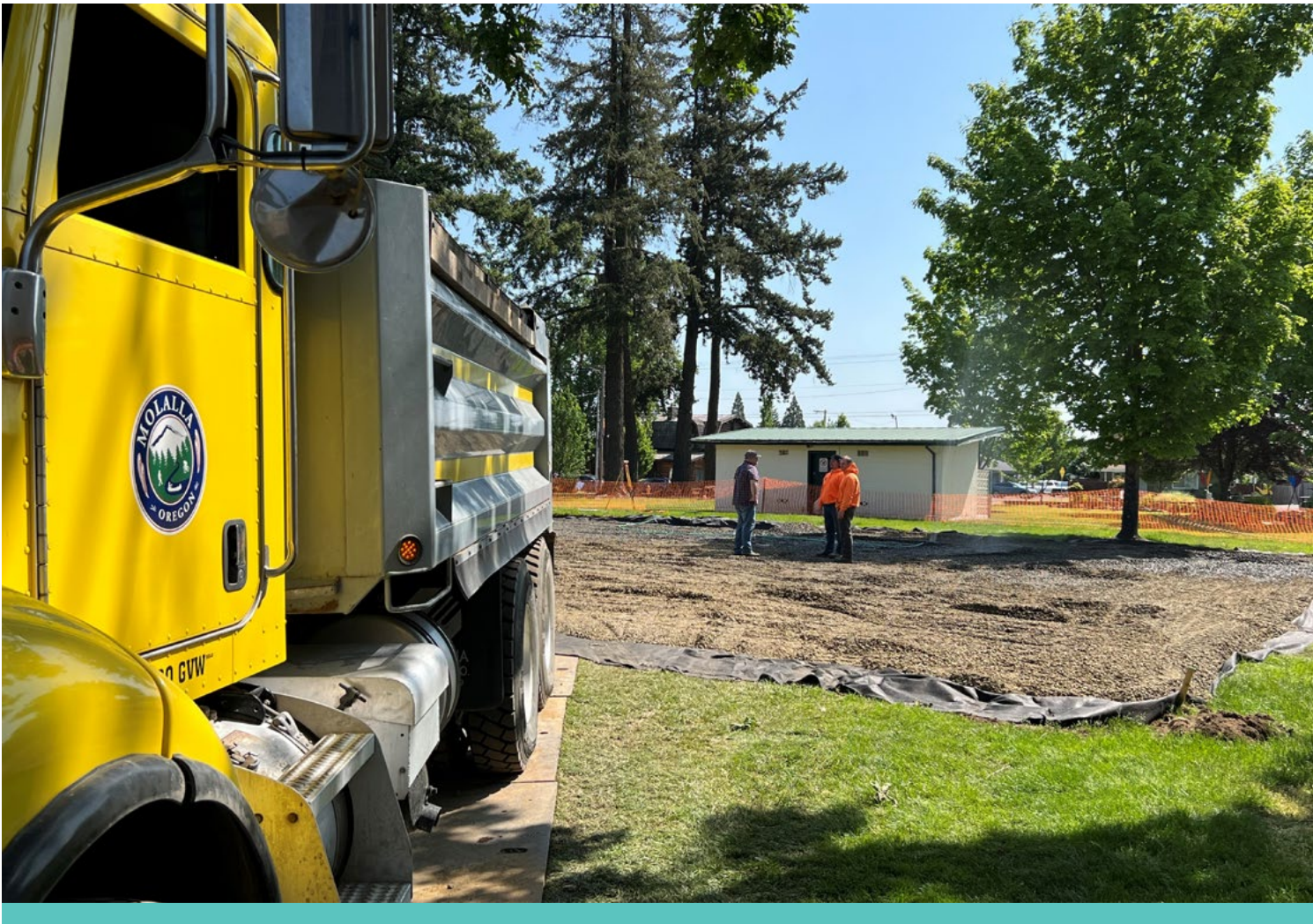
Long Park pickleball court construction
