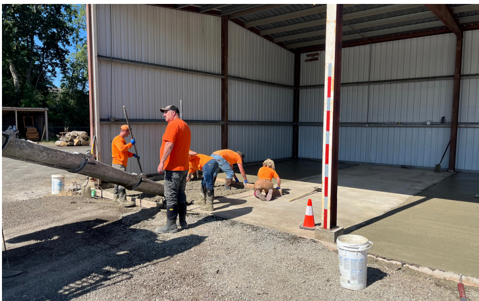
L & ABOVE: CREW POURING & FINISHING CONCRETE AT THE CITY SHOPS
