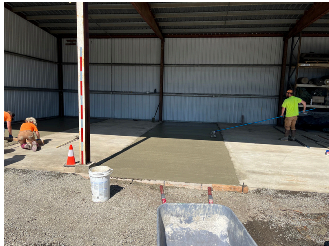
L & ABOVE: CREW POURING & FINISHING CONCRETE AT THE CITY SHOPS
