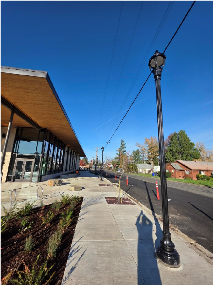
Figure 1- 11.21.2025- New PGE light poles installed
