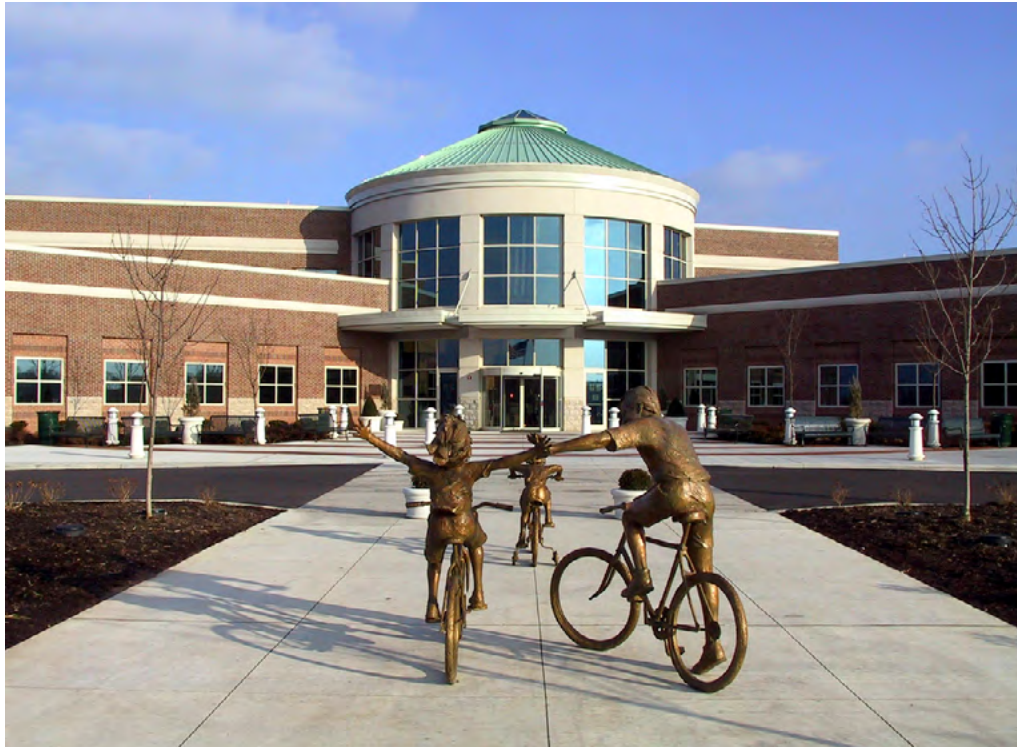
Examples of well-designed building entrances
