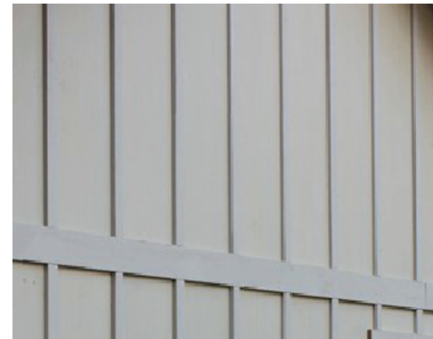
BOARD & BATTEN HARDIE BOARD WITH 1-1/2" CEDAR BATTENS 12" O.C. BATTENS
