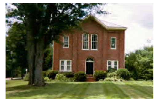
The old school building is located in the Southwest quadrant.
