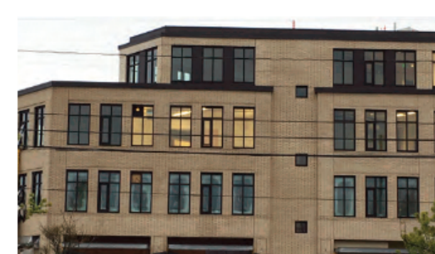
Encouraged Materials: The use of brick, high quality “punched” (recessed) windows, metal awnings and cornices shown above both relate to traditional neighborhood materials and contribute to a feeling of lasting durability
