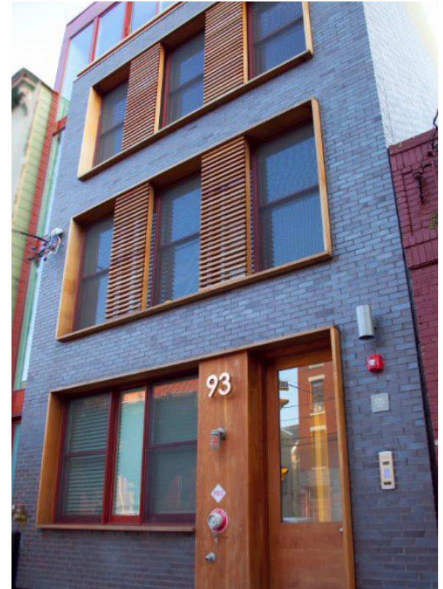
Fig. 21 A contemporary infill development with traditional materials, an innovative approach to historic window proportioning and recessed upper floor (Source: Jorge Mastropietro Architects Atelier)
