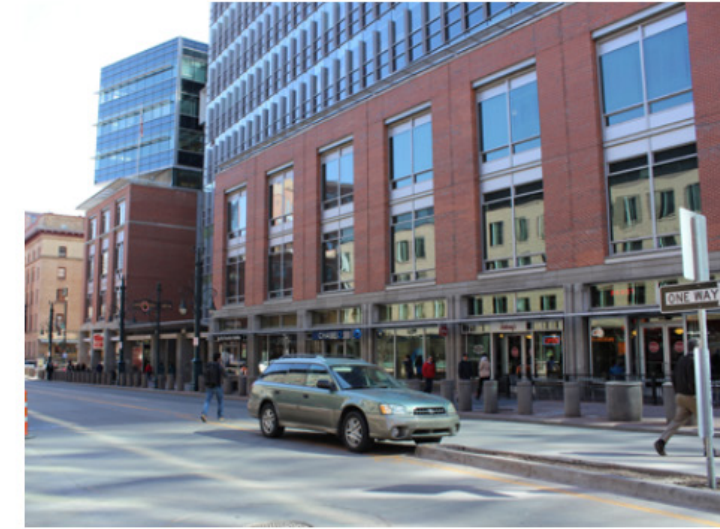
Fig. 12 New construction with appropriate historic references including materiality and facade divisions (Source: City of Boulder)
