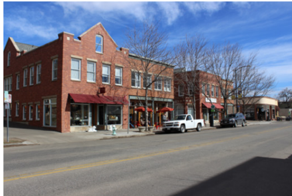
Fig. 10 New construction with compatible material, scale and window proportioning (Source: City of Boulder)
