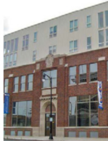
Fig. 7 A non-conforming addition with incompatible materials, massing and window proportioning (Source: National Park Service)
