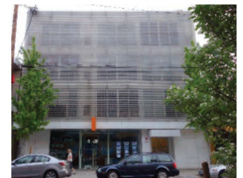
Discouraged Materials: Plastic siding and metal screens were strongly discouraged by community mem-bers in public surveys about design preferences.
