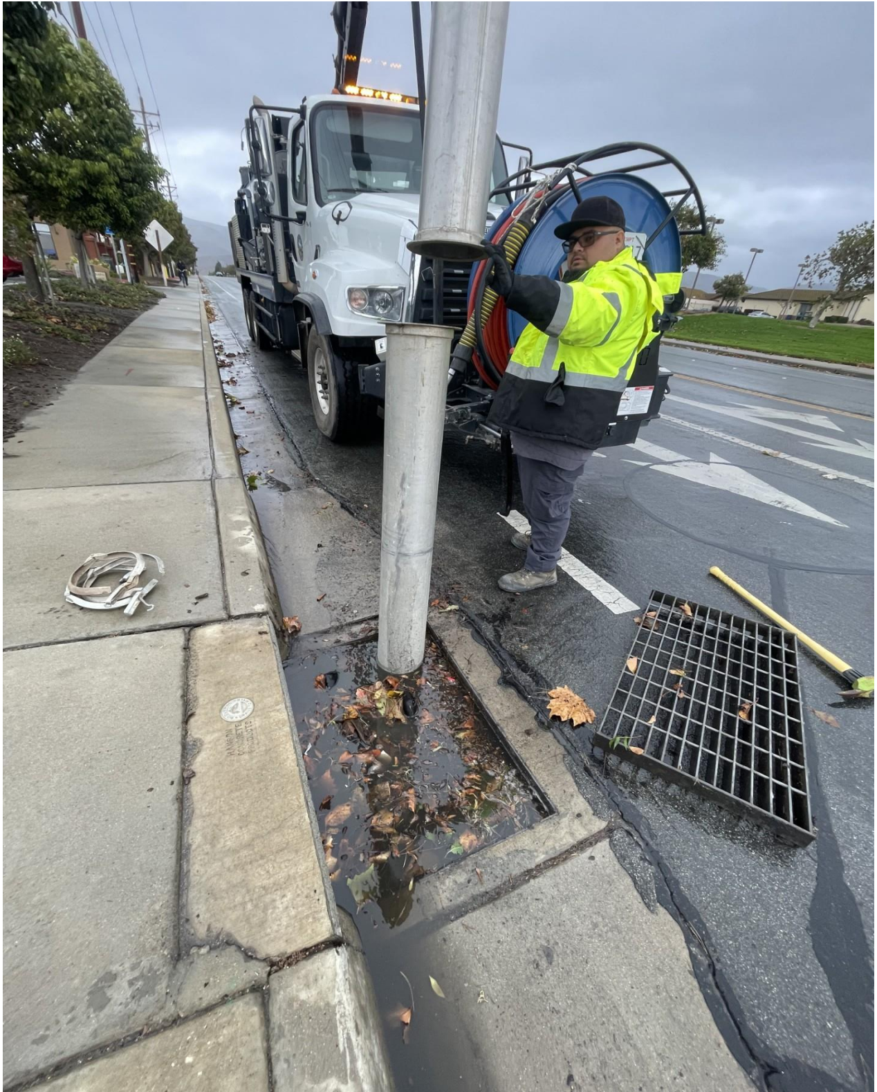
Figure 3 – Storm Drain Cleaning
