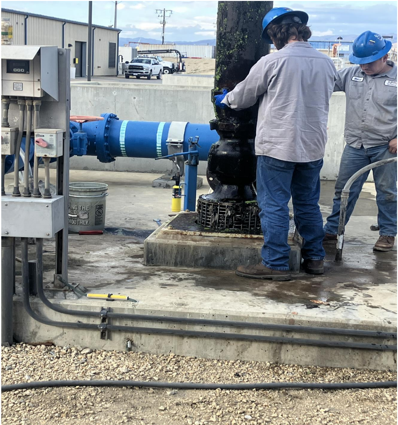
Figure 1 – Extracting E.Q. Pump at WRF
