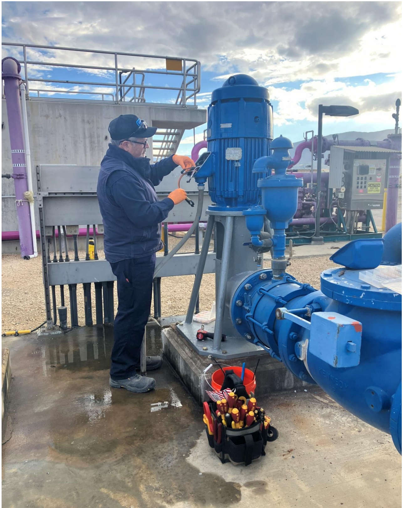
Figure 2 – PW staff rewiring pump at WRF
