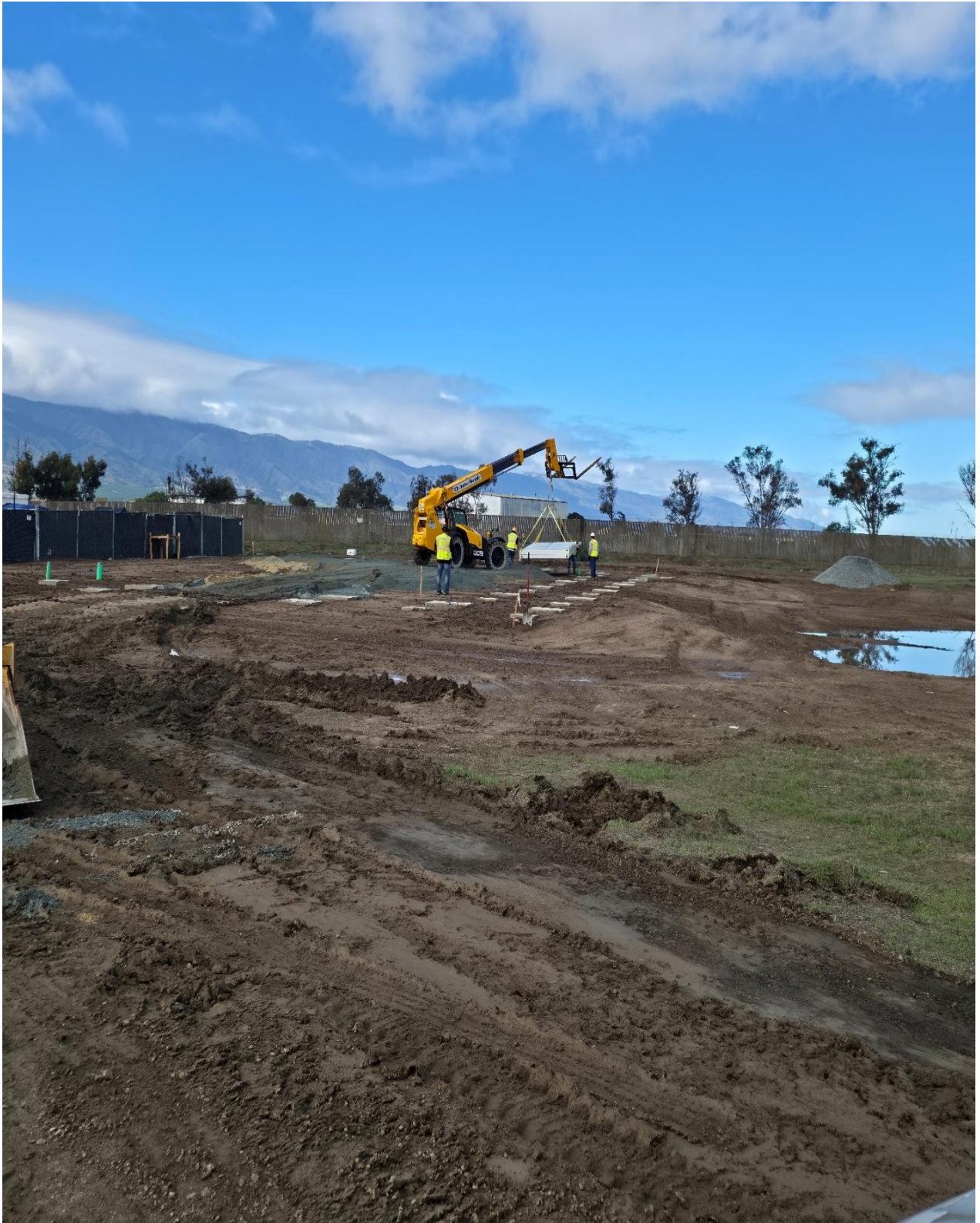
Figure 6-Work at ERF Project
