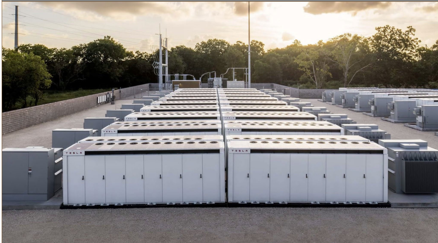
Example of a close-up view of a BESS inside its fenced-in area.
