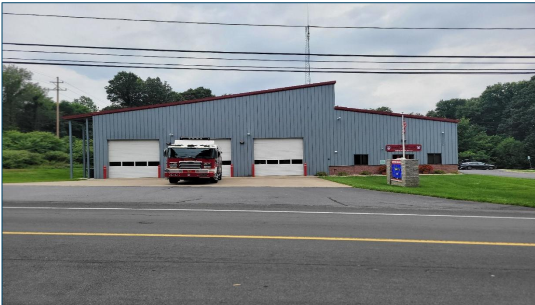
Figure 19 CFR Fire Station 9-1
