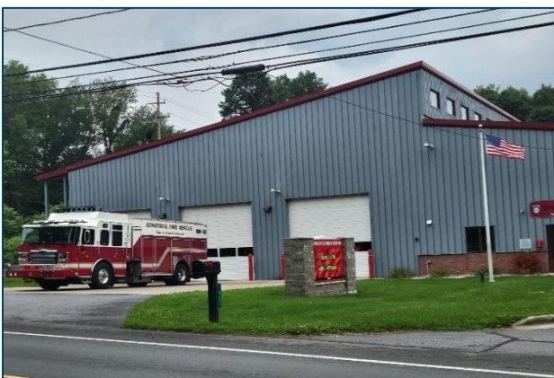
Figure 7 CFR Fire Station #3
