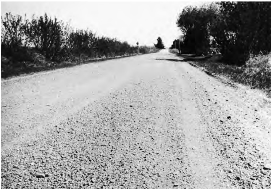
▲ Loose aggregate over most of road. Light grading and compaction during wet weather would improve stability and develop a surface crust.
