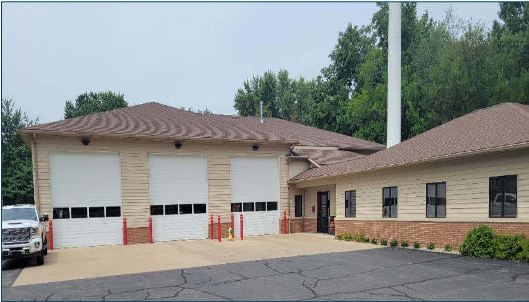
Figure 20 CFR Fire Station 9-2
