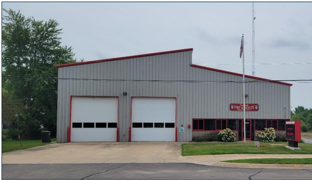
Figure 21 CFR Fire Station 9-3
