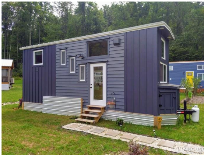
A Movable Tiny Home with skirting installed
