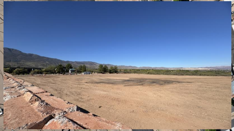
Current site condition — clear & grub complete
