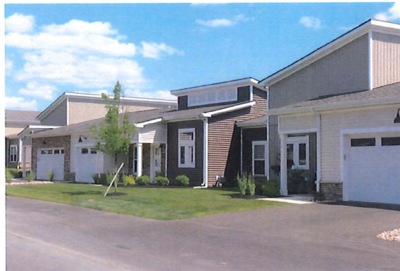
Infill housing located between an older residential area and a shopping center (Redwood / Glenwood Commons) has a contemporary style but is compatible with the scale and character of existing development.
