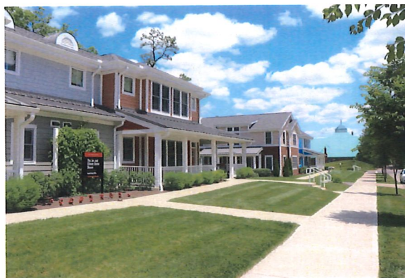
Ohio Wesleyan University's Dittrick House is a redevelopment project that provides duplex-style small living units (SLUs) for students.
