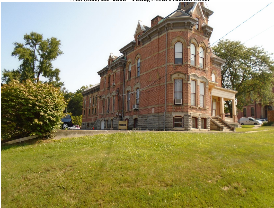
West (Side) Elevation – Facing North Franklin Street
