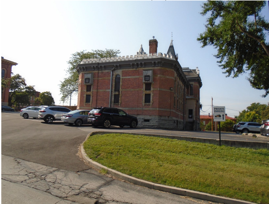
Historic Jail & Sheriff Residence – North (Rear) Elevation – August 2023
