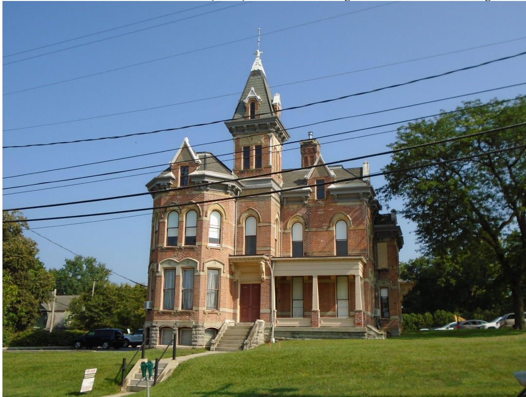
Historic Jail & Sheriff Residence – South (Front) Elevation - Fronting West Central Avenue - August 2023
