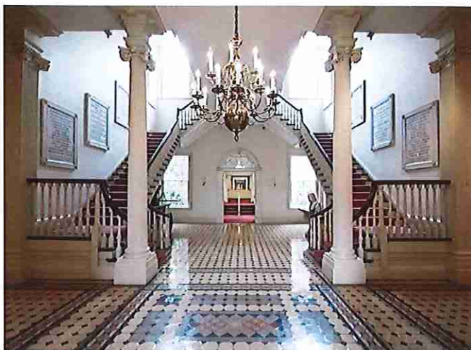
Great Hall with hidden sprinkler heads
