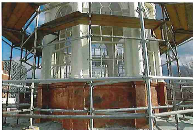
East cupola copper cladding and window restoration in progress.
