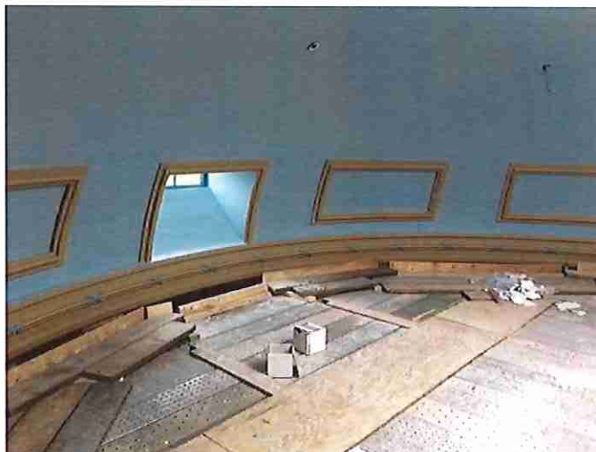
Surgical Amphitheater ceiling during fire protection installation.
