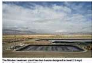
The Minden treatment plant has two basins designed to treat 1.5 mgd average flow in about 100,000 gal.
